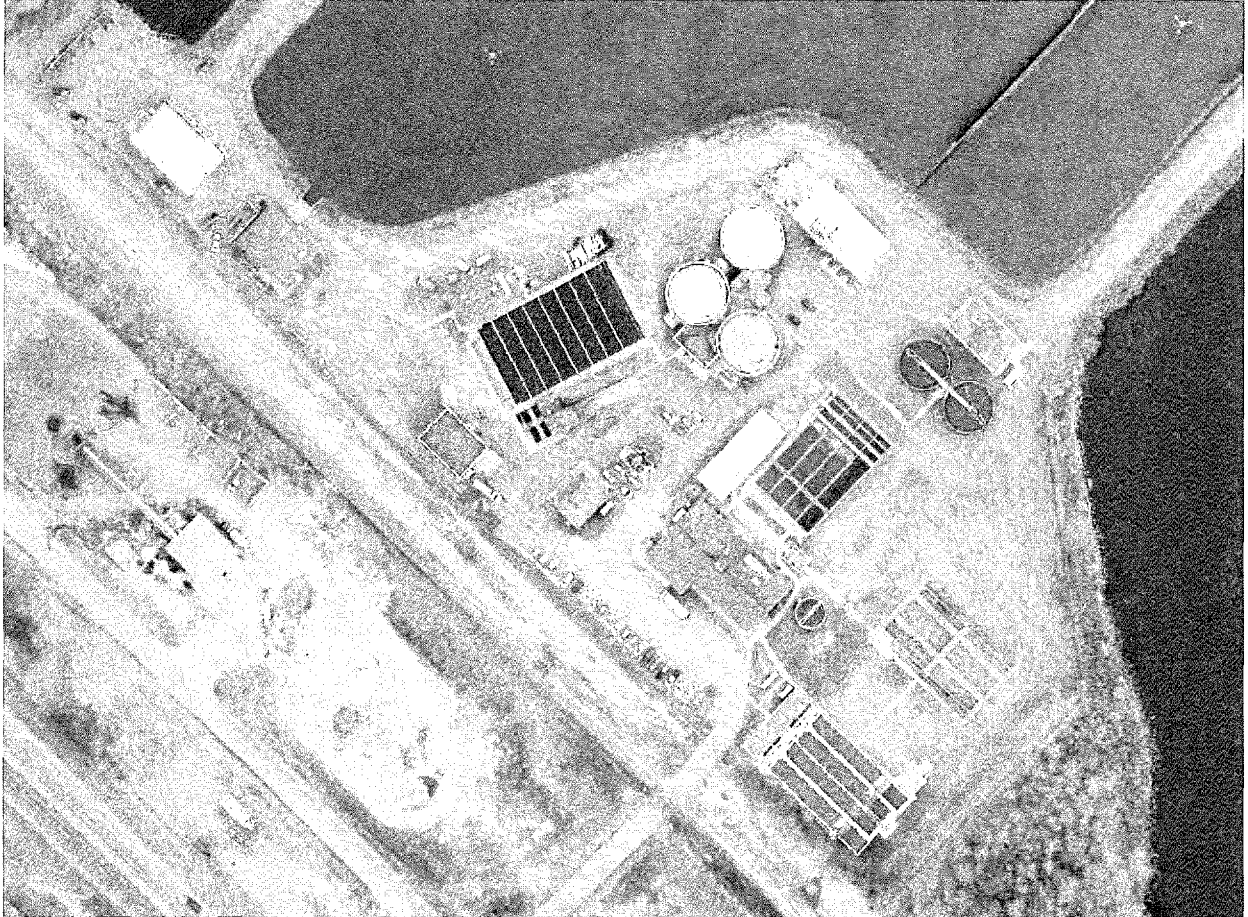
Figure 1 City of Superior Wastewater Treatment Facility
