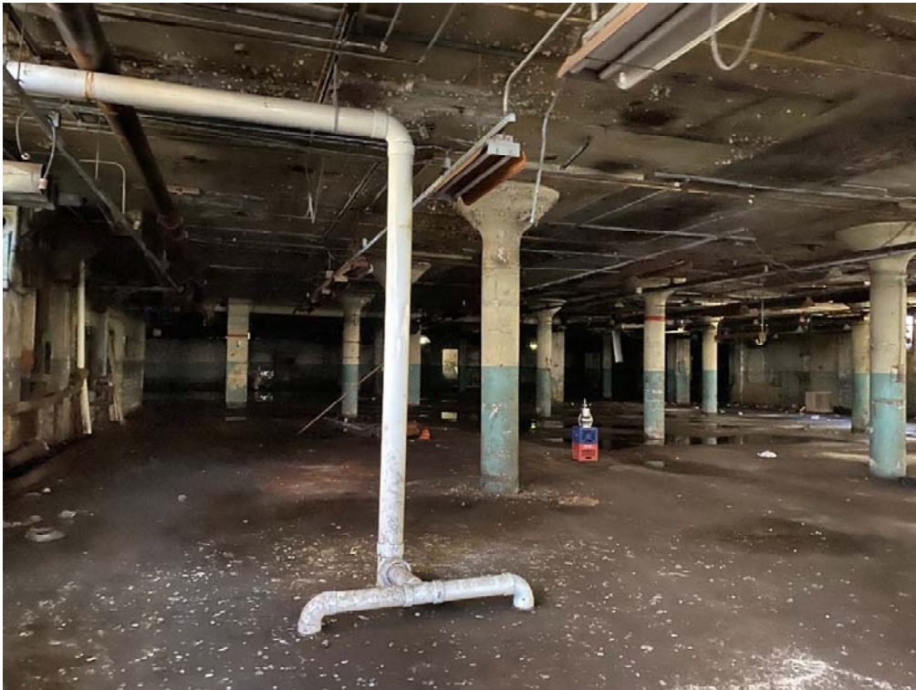
Level 1 – Building 2B (view to East)
