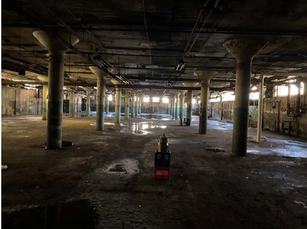
Level 1 – Building 2A (view to West)
