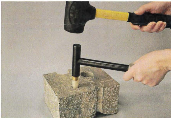
Figure 2. Installing the FLX-VP™
