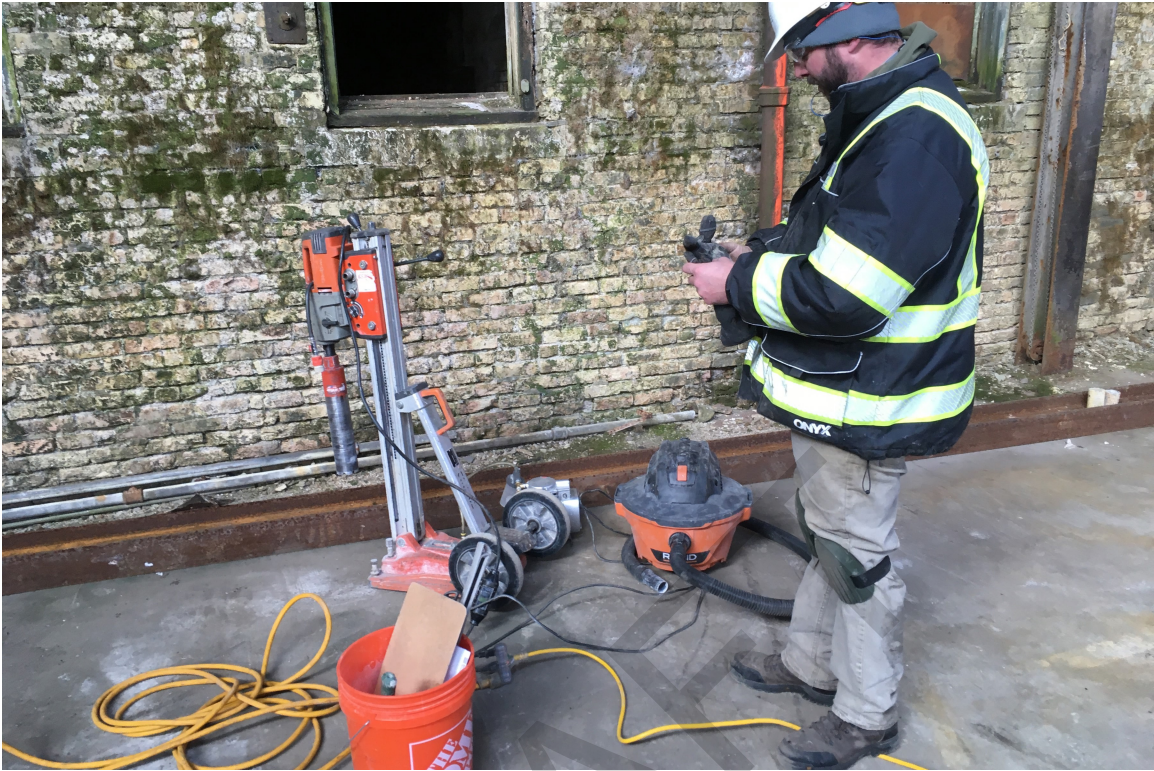
Photograph 1. Installation of PFE VE#5
