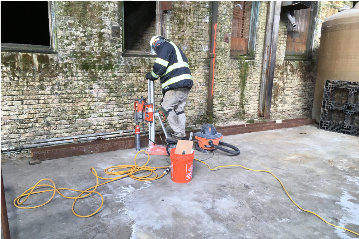
Photograph 2. Installation of PFE VE#5
