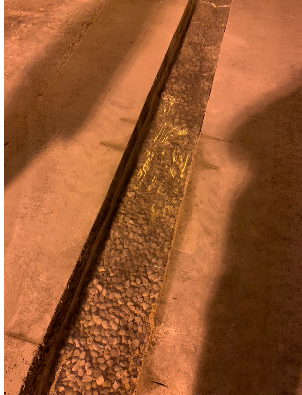
Final Grade of Underground Pipe w/ Vapor Barrier
