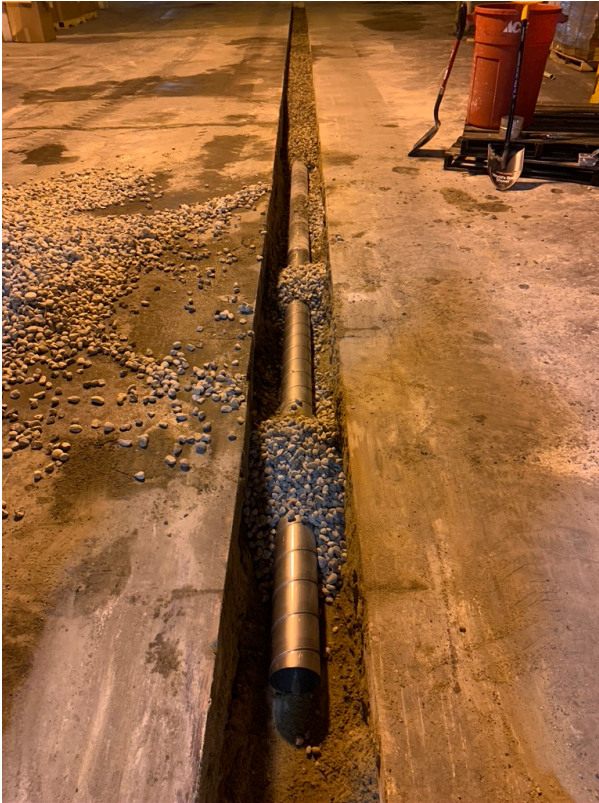
Backfilling Underground Pipe
