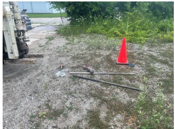
Photo #6 Soil boring and temporary groundwater monitoring well P-6 facing south.
