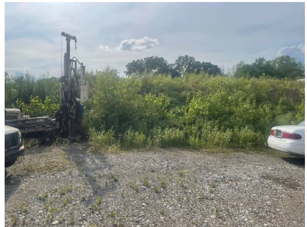
Photo #10 Soil boring and temporary groundwater monitoring well P-10 facing west.
