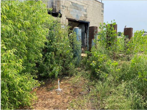
Photo #13 Soil boring and temporary groundwater monitoring well P-13 facing southeast.
