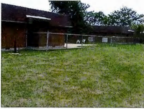
Photo 1 – Health Care Center – Pre-Demo
