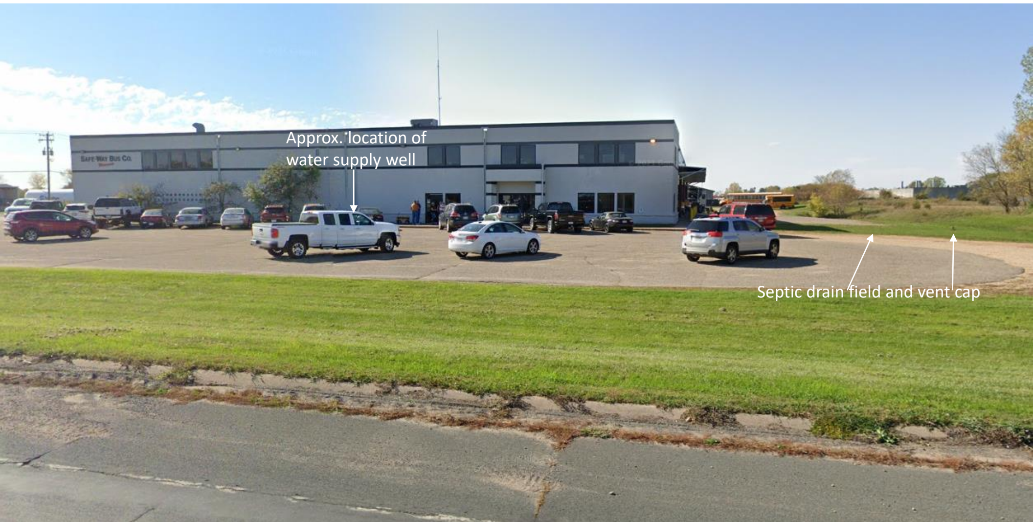
Looking west from County. Rd. U at the eastern side of the facility.
