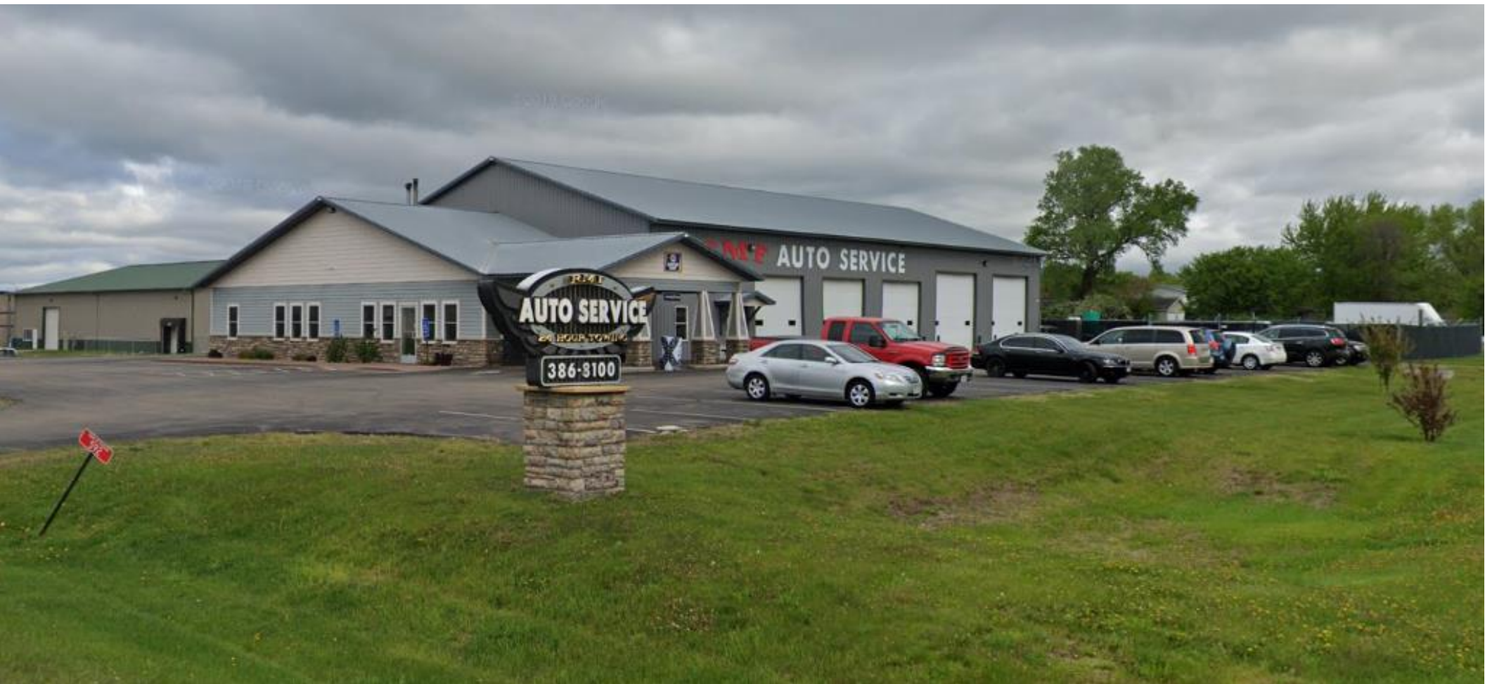
Looking northwest from Schommer Dr. at the south and east sides of the facility.
