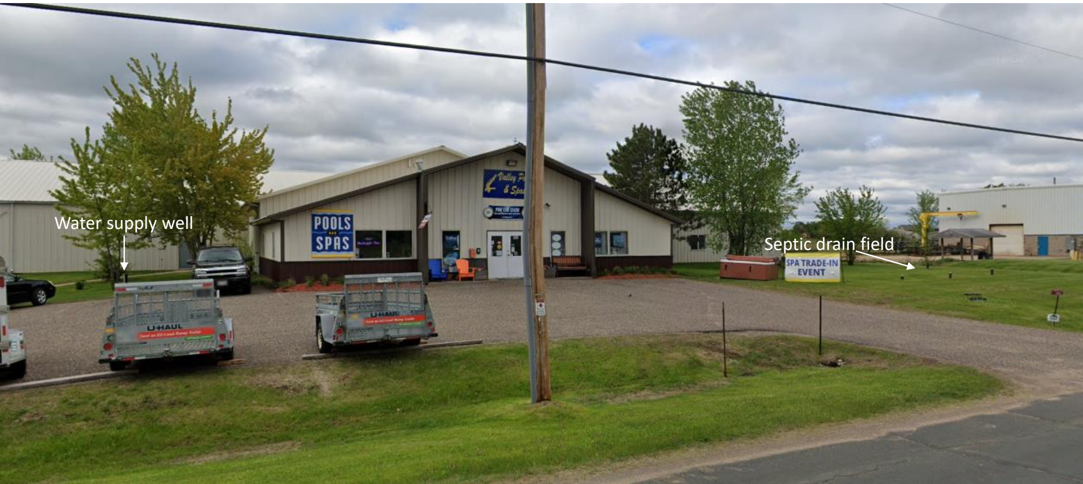
Looking south from Schommer Dr. at north side of the facility.
