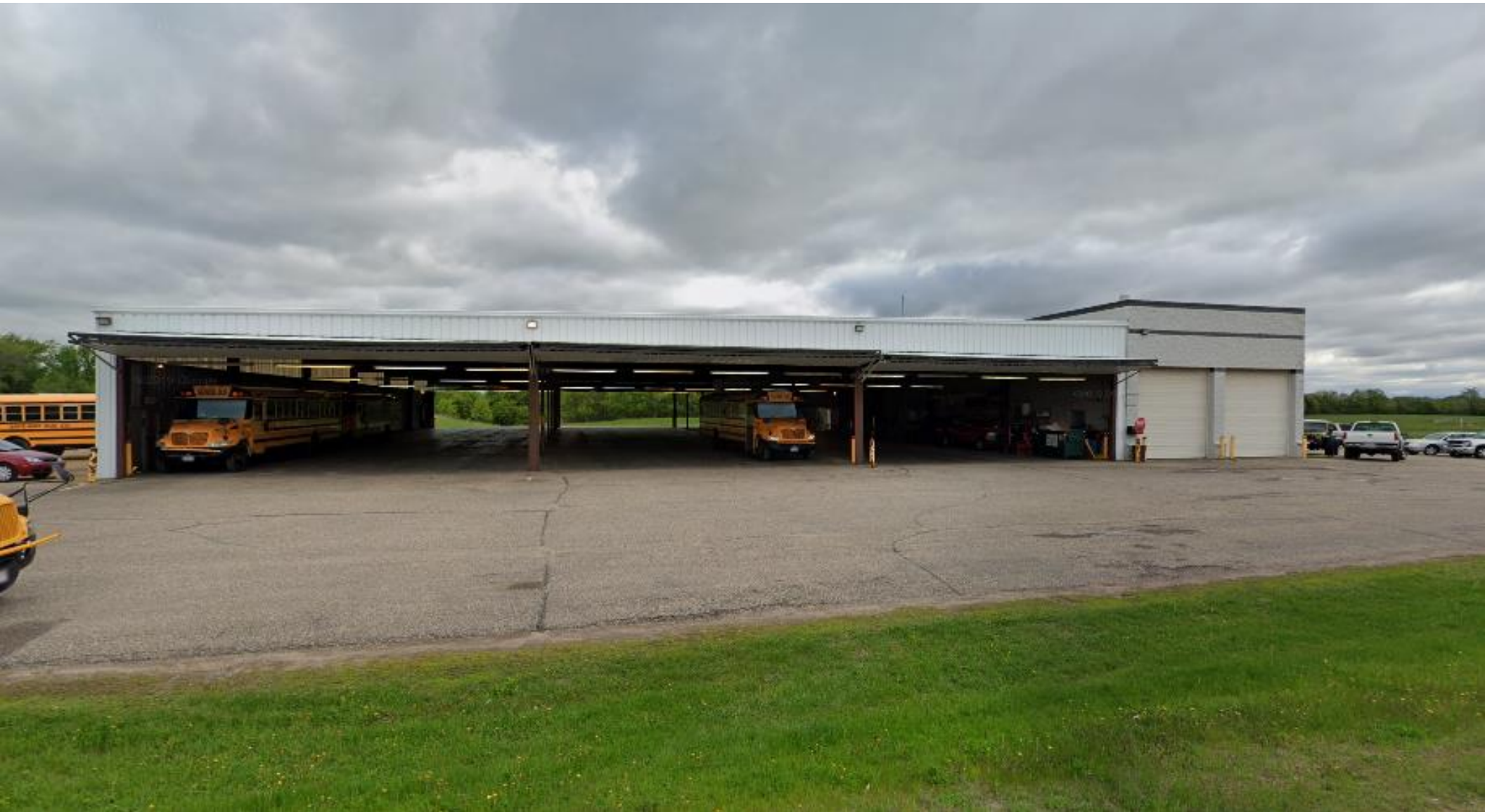
Looking north from Schommer Dr. at the southern side of the facility.
