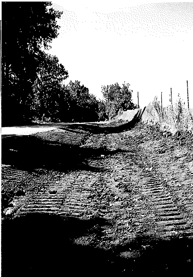
Photo #32 Completed clay compaction and topsoil replacement - South Perimeter Ditch
