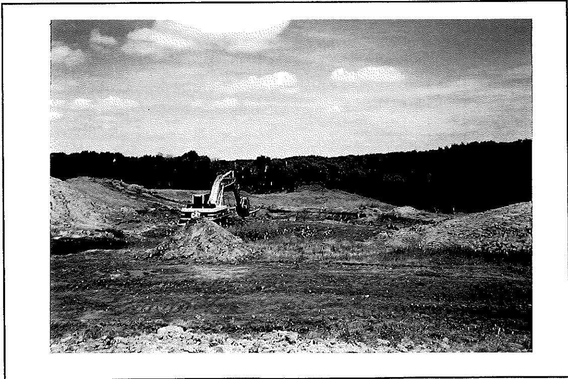
Photo #6 Spreading solid waste excavated from uncapped areas - Landfill Cap
