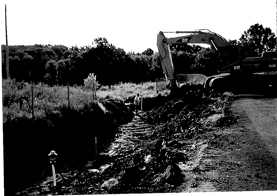
Photo #31 Removal of surface soils near eastern end of ditch - South Perimeter Ditch
