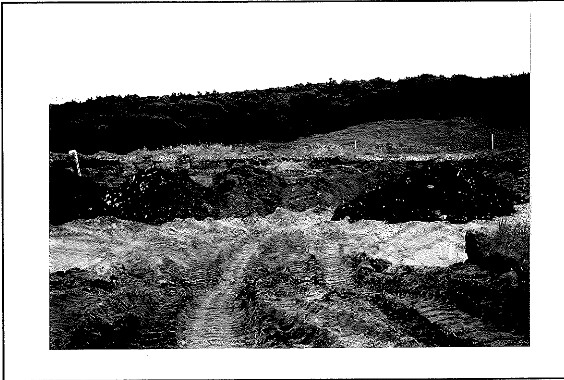
Photo #9 Stockpiling solid waste in subsidence area - Landfill Cap
