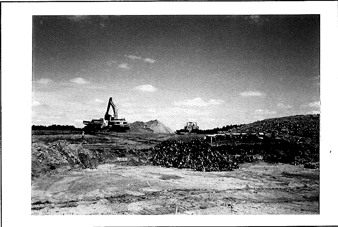
Photo #7 Preparing to spread solid waste in subsidence area - Landfill Cap
