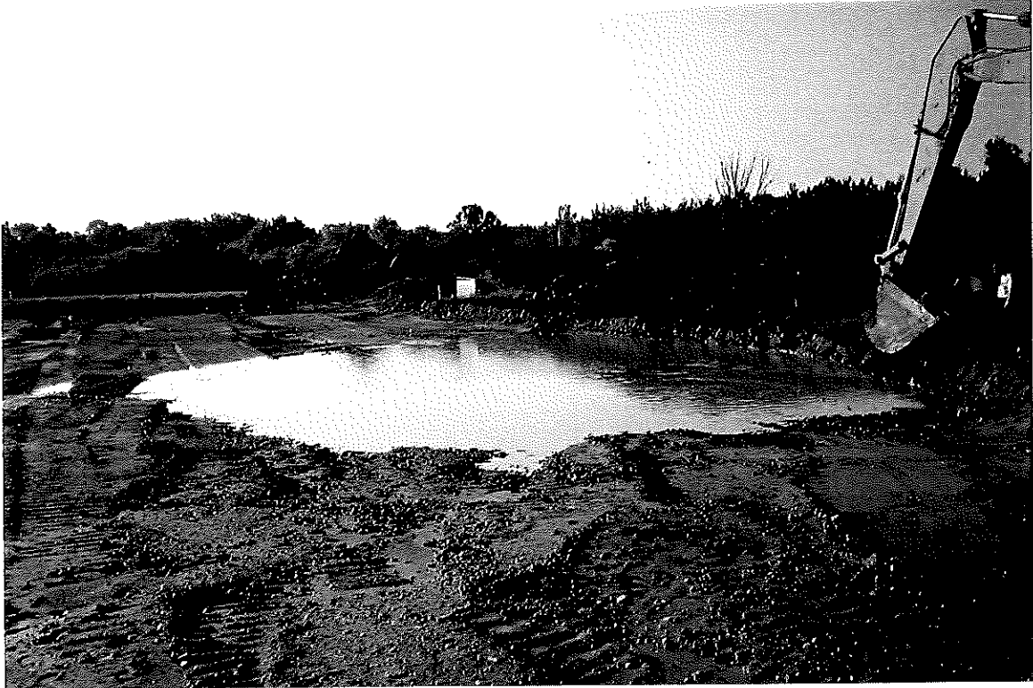
Photo #3 Installing submersible pump for rainwater removal - Landfill Cap
