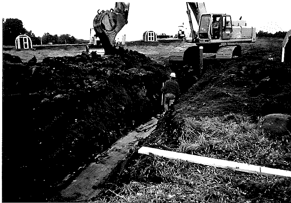
Photo #24 Trenching to LEW-1 for lateral pipe connection - Landfill Cap
