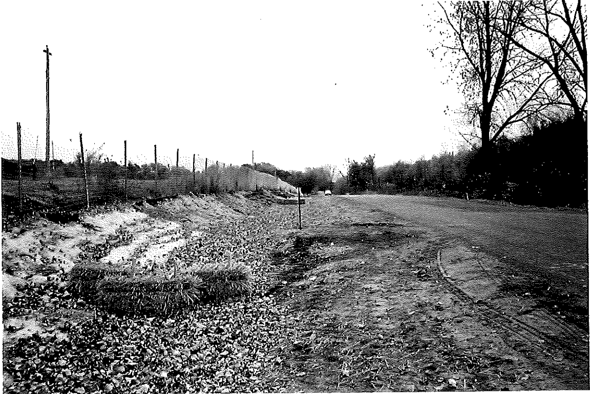
Photo #33 Seeding and mulching and fence restoration complete - South Perimeter Ditch
