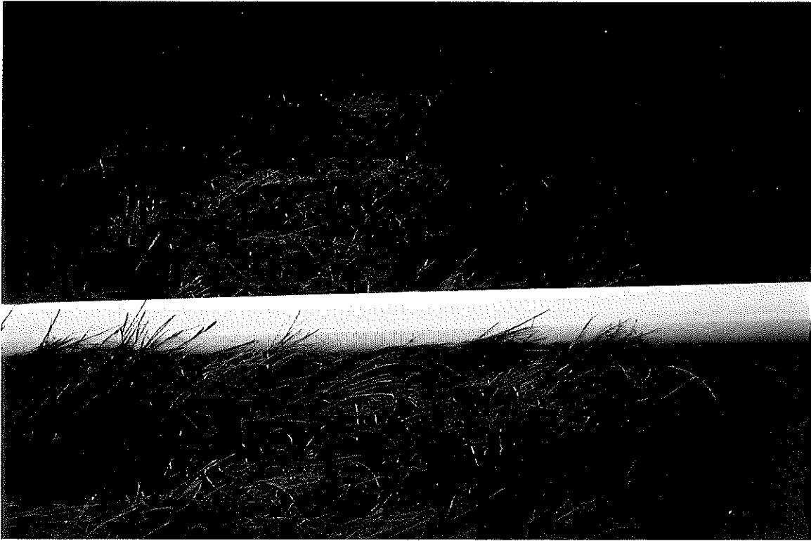
Photo #15 Gas/Leachate extraction well screen - Landfill Cap
