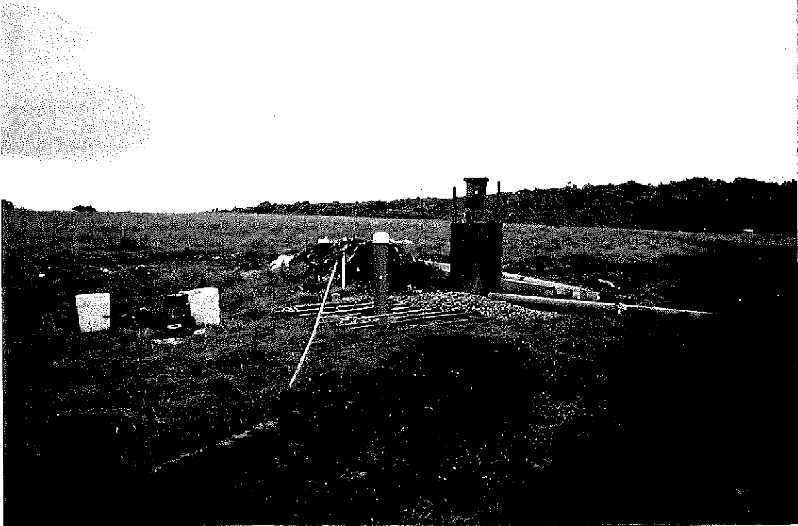
Photo #16 GEW-19 installation and backfill complete - Landfill Cap
