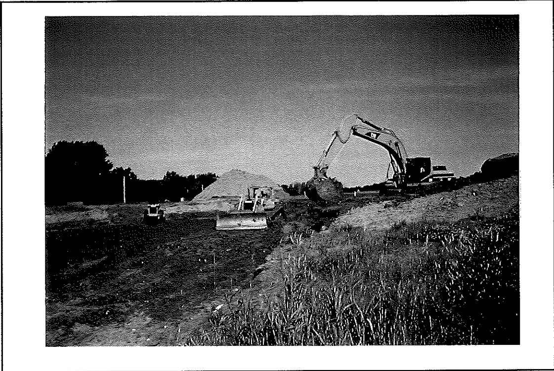
Photo #11 Placing and compacting clay - Landfill Cap
