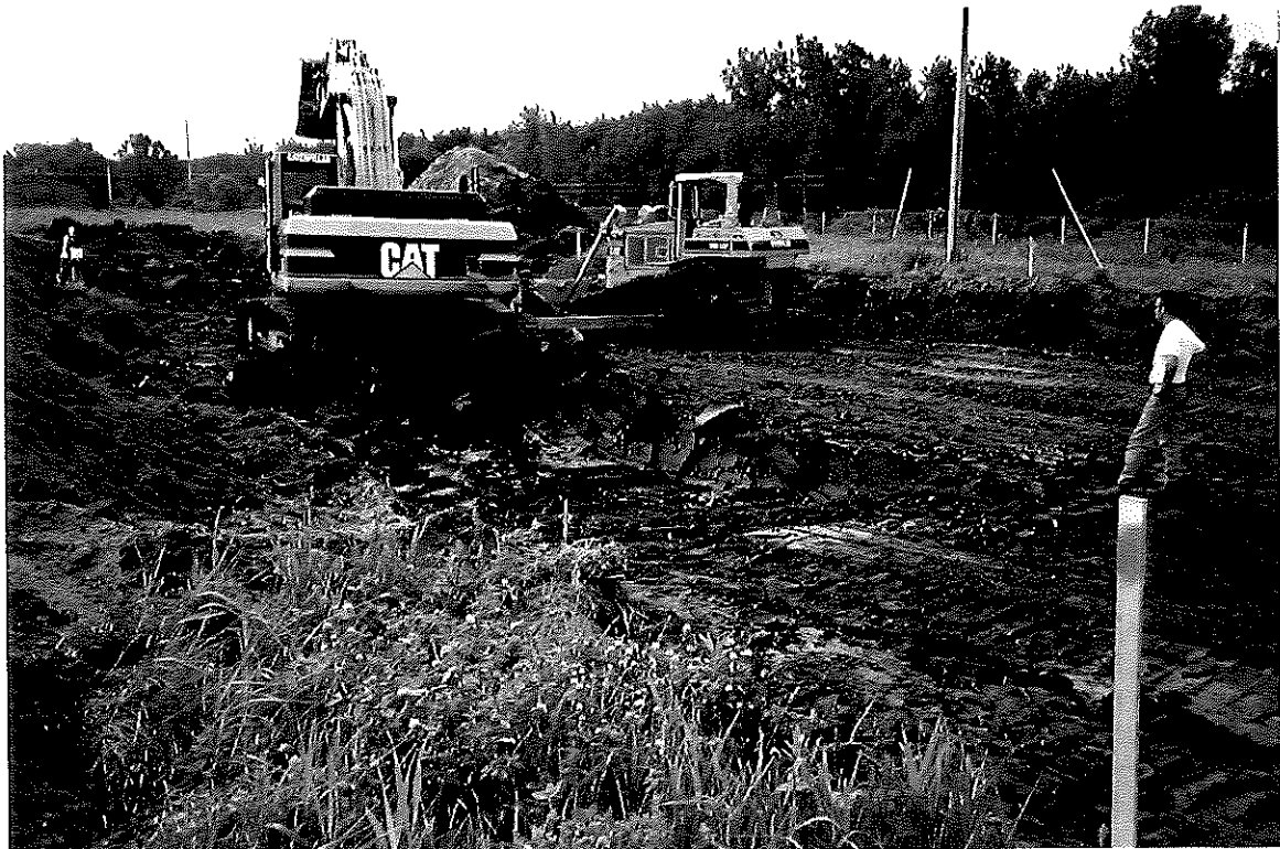
Photo #4 Stripping clay from subsidence areas - Landfill Cap
