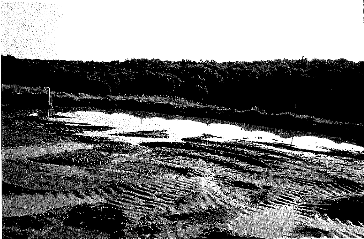
Photo #2 Rainwater collecting in subsidence area - Landfill Cap
