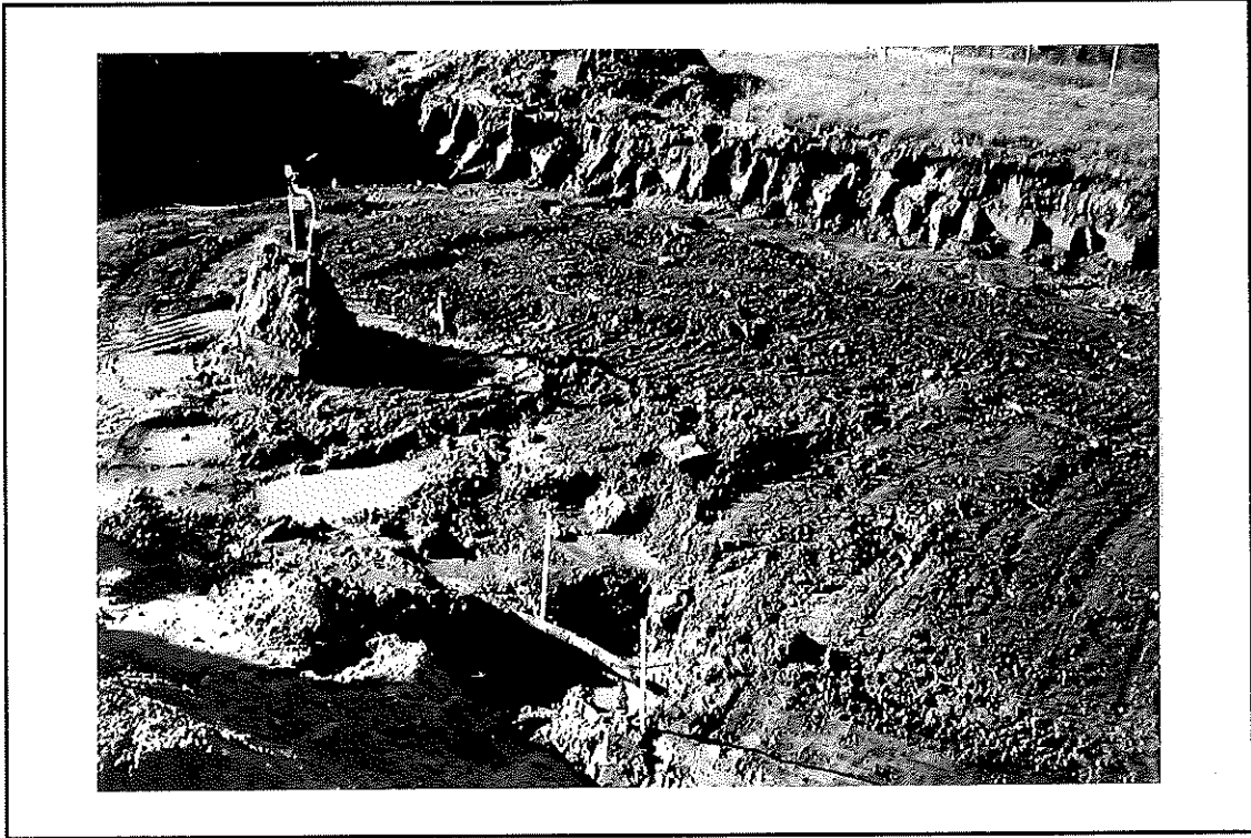
Photo #5 Broken lateral piping to GEW-13 - Landfill Cap
