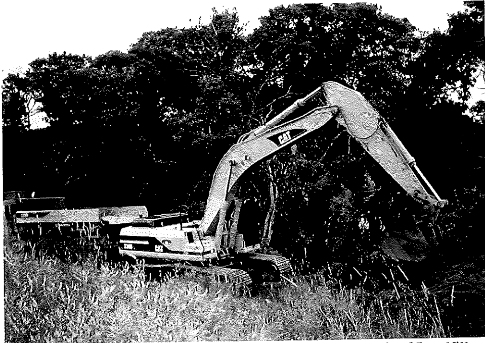
Photo #13 Excavating uncapped solid waste area - north of Landfill Cap
