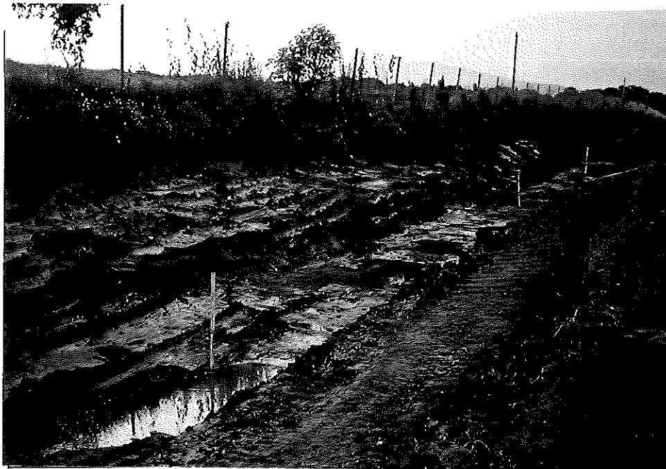
Photo #30 Removal of surface soils in western ditch complete - South Perimeter Ditch
