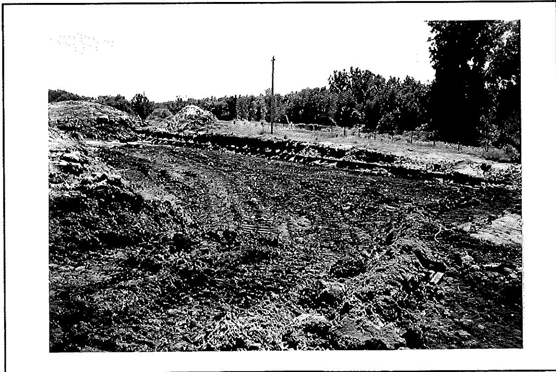
Photo #10 Spreading clay over solid waste - Landfill Cap
