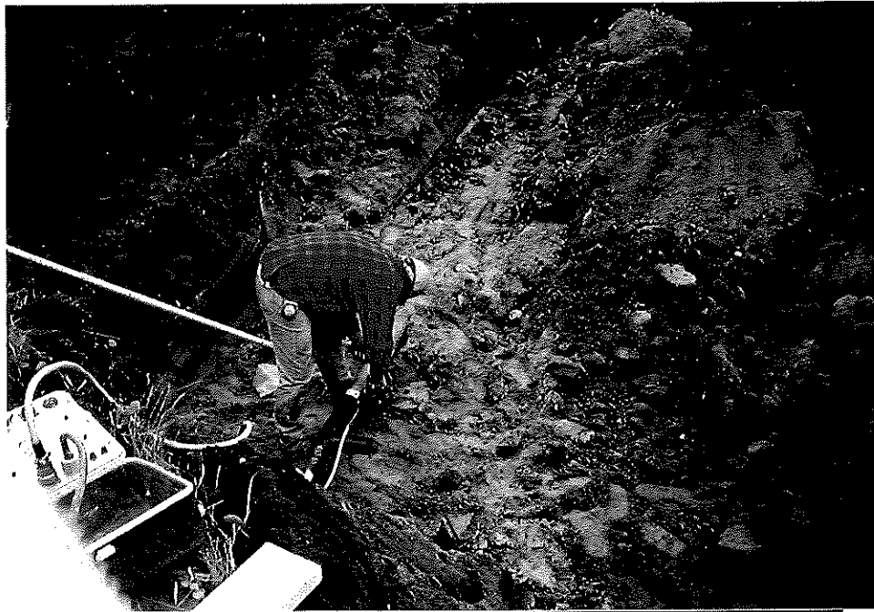
Photo #23 Adding tee to existing lateral piping for connection to new well- Landfill Cap
