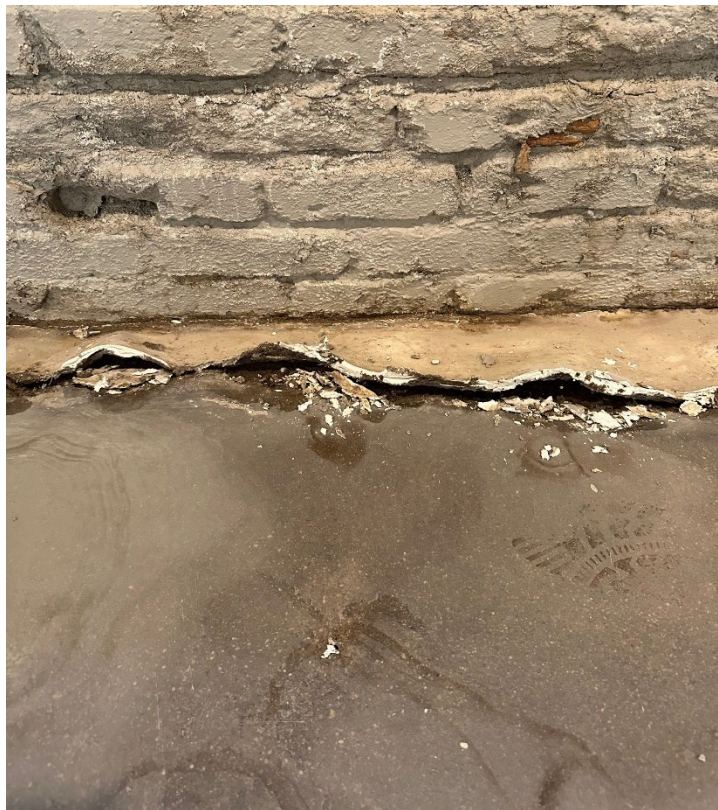
Photo 34 - A closer look at the wall and flooring
