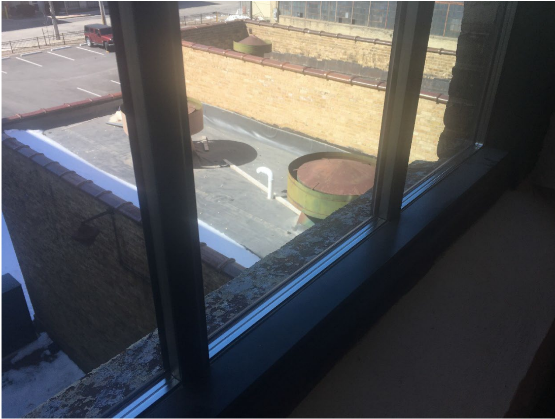
Photo 39 – Fan outlet for North Mechanical Room and Powerhouse
