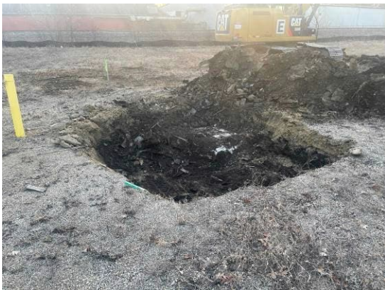
Photo #9 Photograph of soil excavation and disposal of Area 2.
