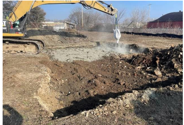
Photo #2 Photograph of soil stabilization of excavation Area 1 facing northeast.
