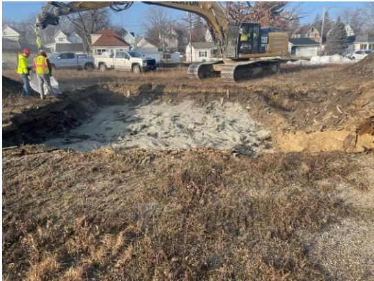
Photo #7 Photograph of soil stabilization of excavation Area 1.
