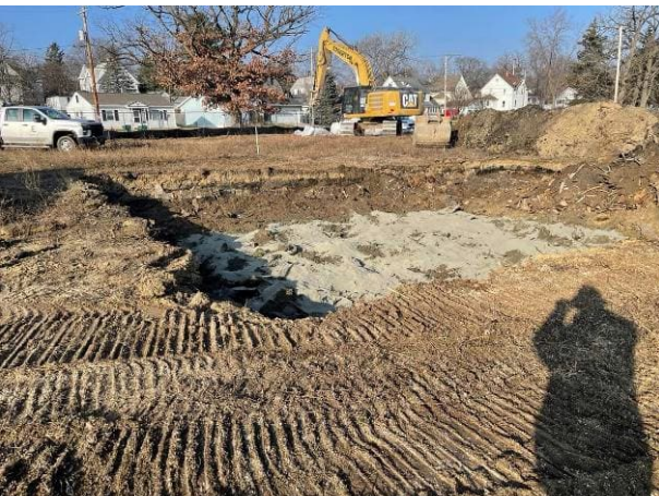
Photo #5 Photograph of soil stabilization of excavation Area 1 facing west.
