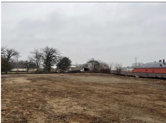
Photo #11 Photograph of backfilled soil excavation Area 1.
