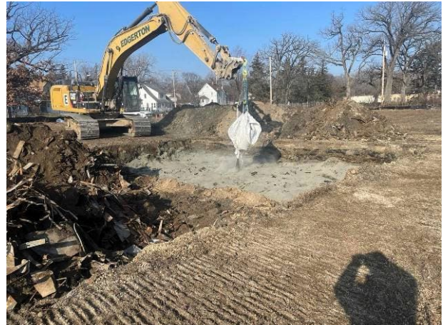
Photo #4 Photograph of soil stabilization of excavation Area 1 facing northwest.
