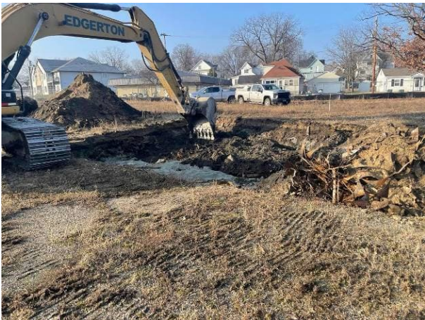
Photo #3 Photograph of soil stabilization of excavation Area 1 facing southwest.
