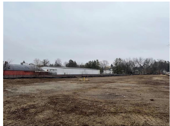
Photo #12 Photograph of backfilled soil excavation Area 1 and 2.
