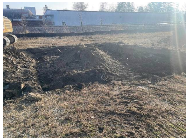
Photo #6 Photograph of soil stabilization of excavation Area 1 facing east.
