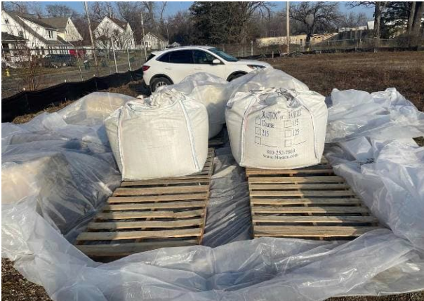
Photo #1 Photograph of Blastox stabilization agent used within excavation Areas 1 and 2.
