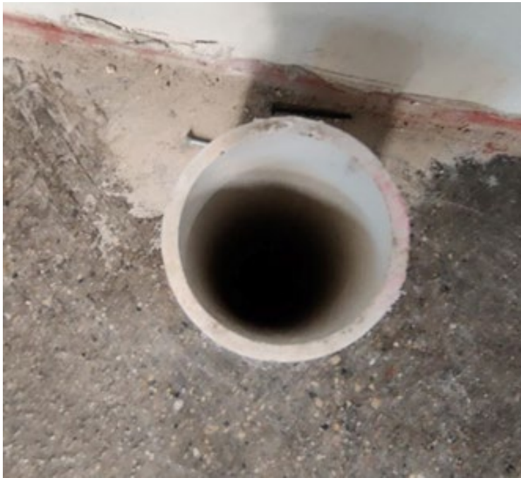
Photo 11: Unit 1052 – Seal open pipe
