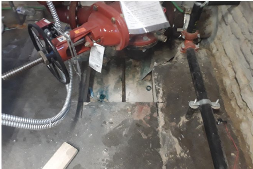
June 1, 2023 - Rebar Installed Under Mechanical Room Cut
