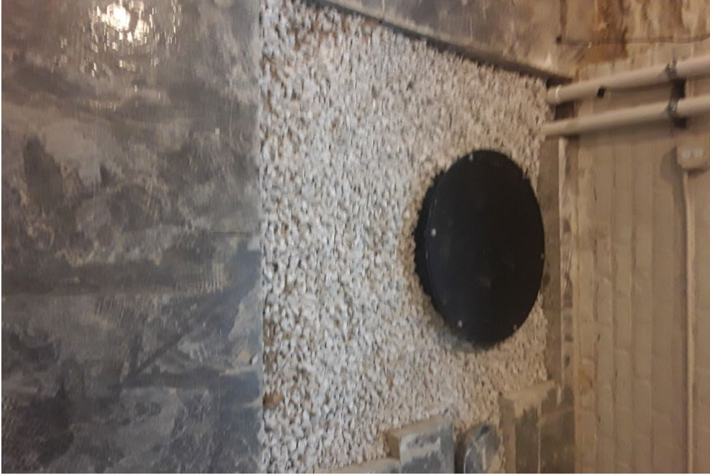
May 30, 2023 - Sump in Unit 1042
