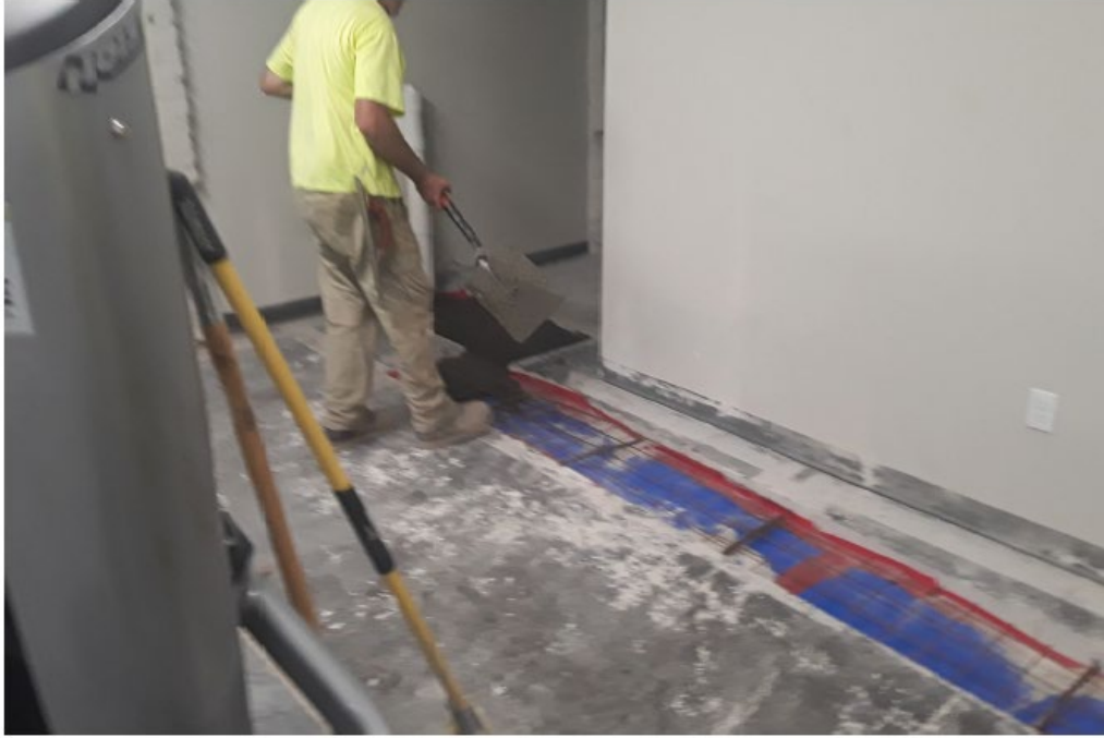
June 1, 2023 - Concrete Sealing in Fitness Room
