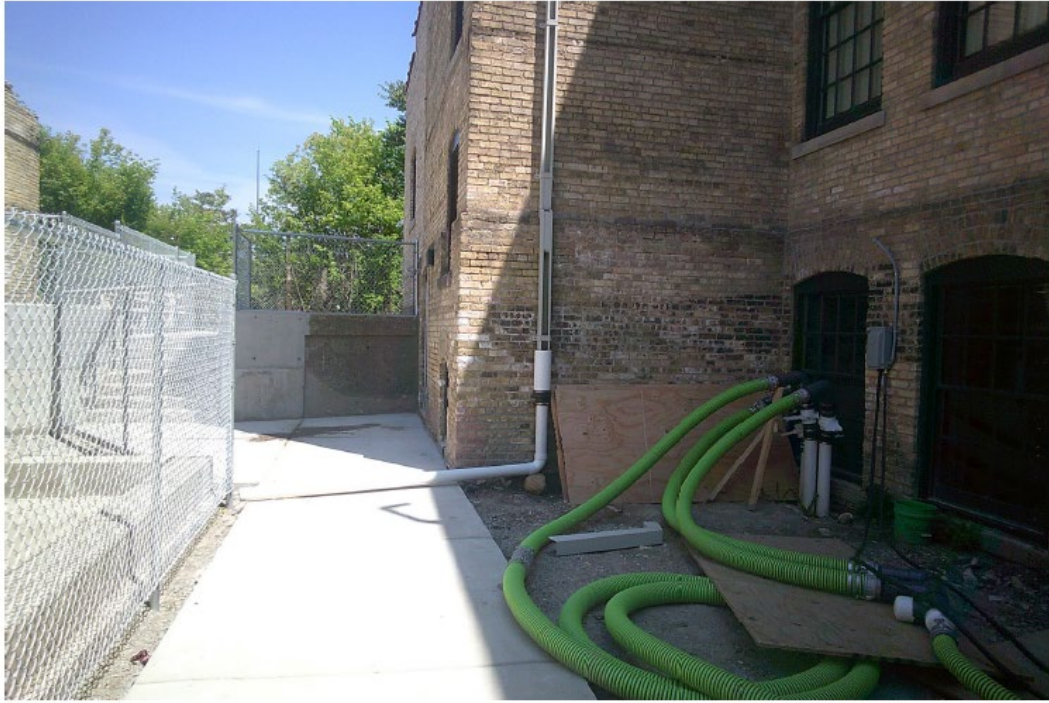
June 2, 2023 - Temporary Redirection of Downspout Discharge
