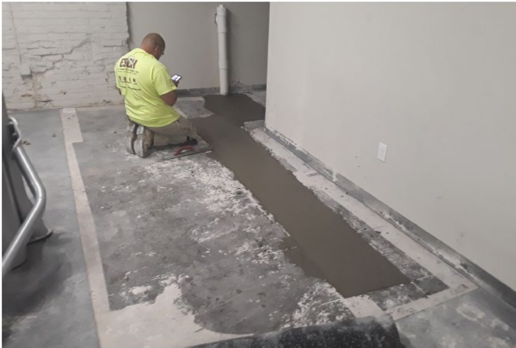
June 1, 2023 - Concrete Sealing of Floor in Fitness Room
