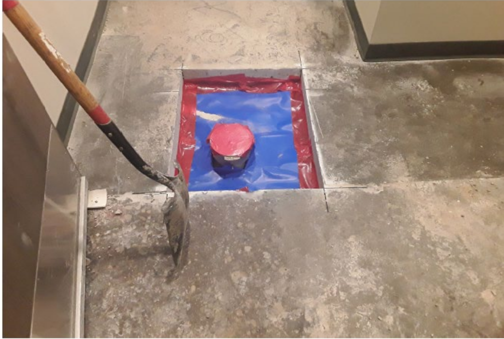
June 1, 2023 - Vapor Barrier Around Inspection Port in Unit 1025
