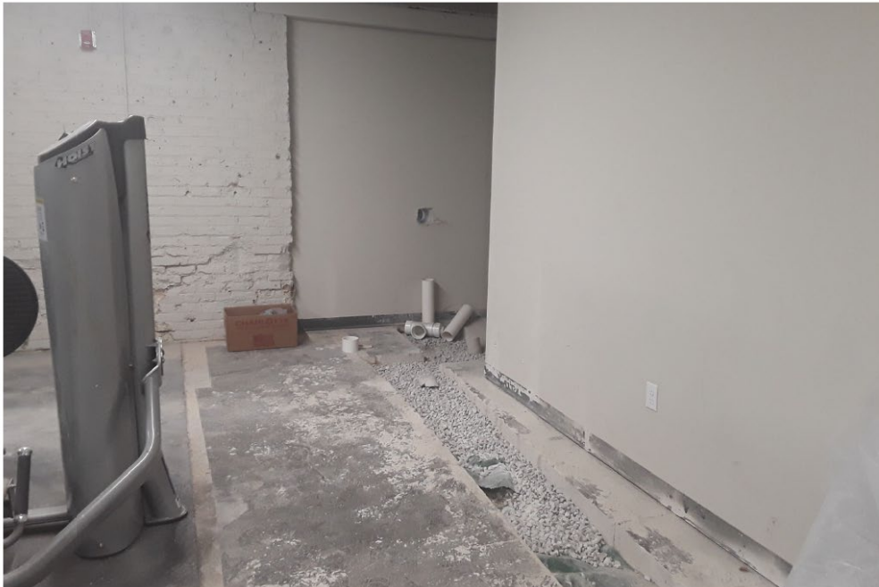
May 30, 2023 - Hole Cored for Piping in Fitness Room
