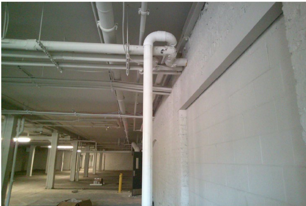
June 2, 2023 - Completed Piping Hookup to Outlet Pipe
