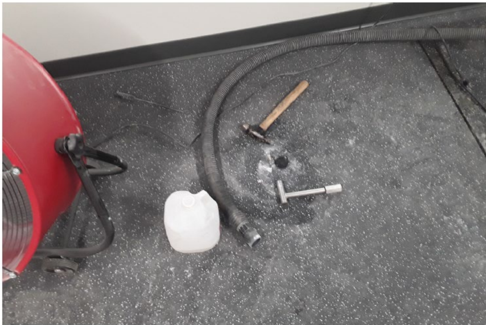
May 31, 2023 - Installed Vapor Pin in Fitness Room
