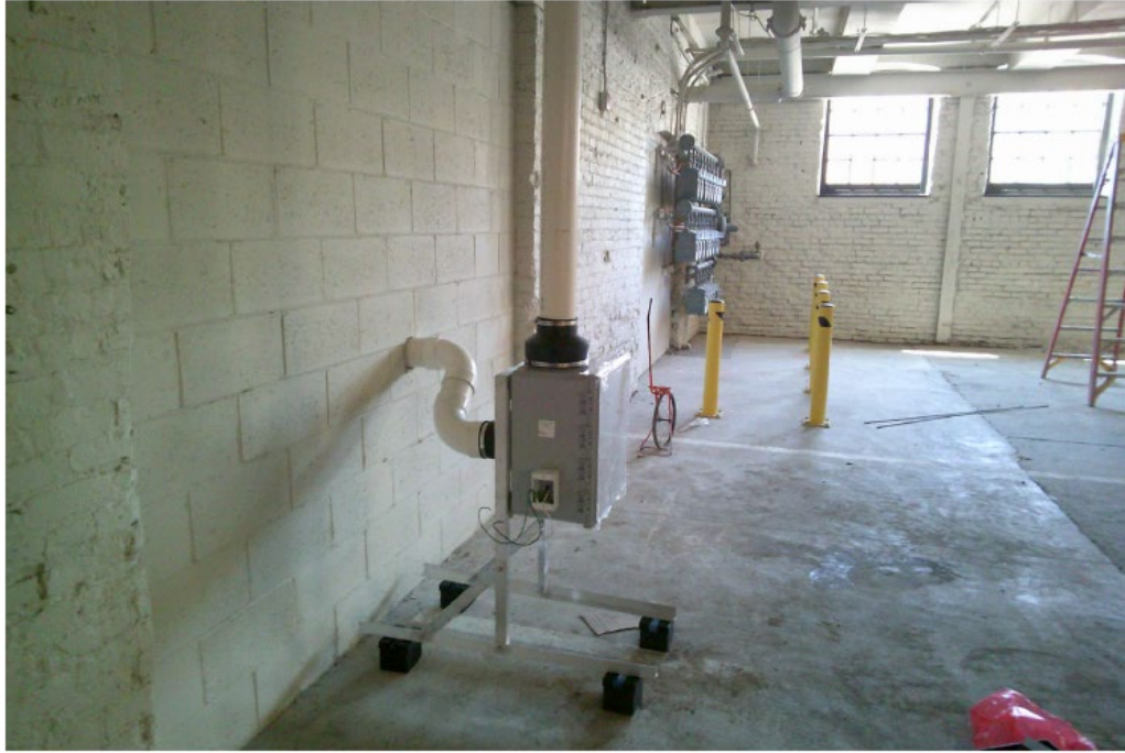
June 2, 2023 - OBAR Fan Hooked Up to Outlet Piping
