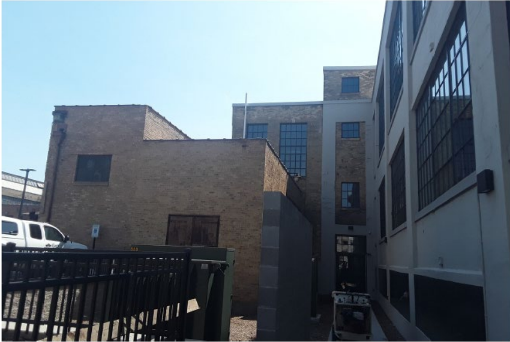
June 1, 2023 - Power House / Mechanical Room Vent Line Above Roof Line
