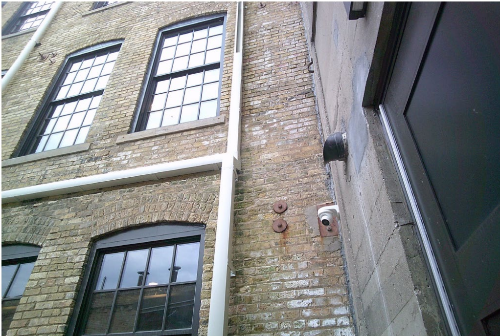
June 6, 2023 - Rerouted Gutters
