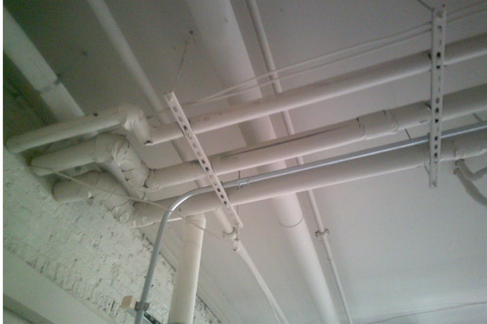
June 5, 2023 - Installed Ceiling Conduit to Obar Fan by Roman Electric
