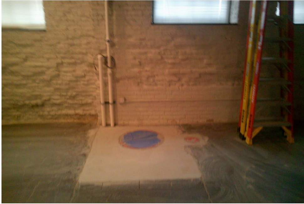
June 5, 2023 - Sump in Unit 1042 - Plumbing Completed
