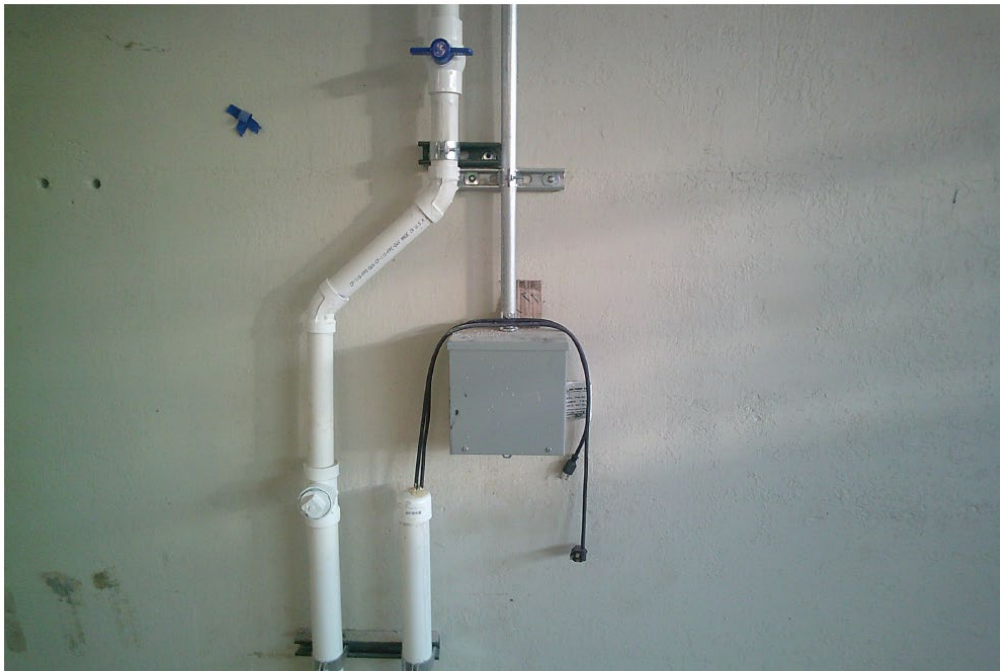
June 5, 2023 - Horner Construction Completed Northern Garage Sump with Plugs
