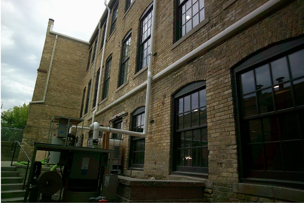
June 6, 2023 - Rerouted Gutters
