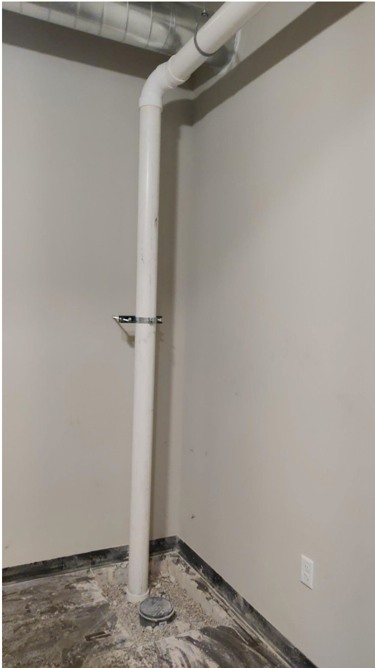
Picture 4 - Preparation for Additional Blower at Access Point 1
