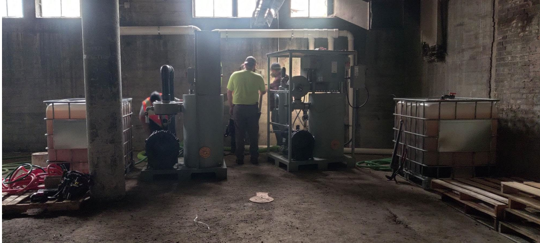
Picture 1 – Installation of 1 Permanent Blower
