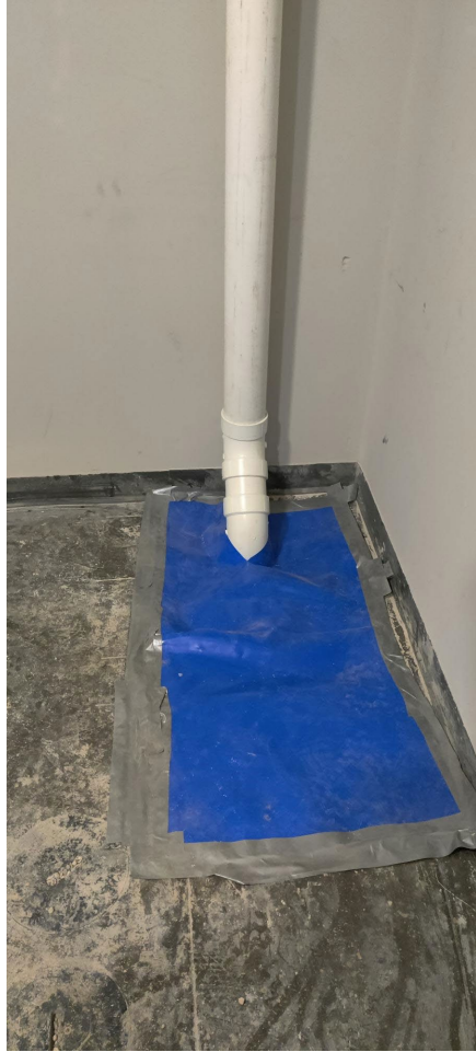
Picture 3 – Sealing of Access Point of Blowers 7
