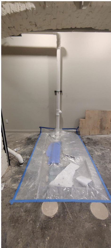
Picture 2 – Sealing of Access Point of Blowers 6
