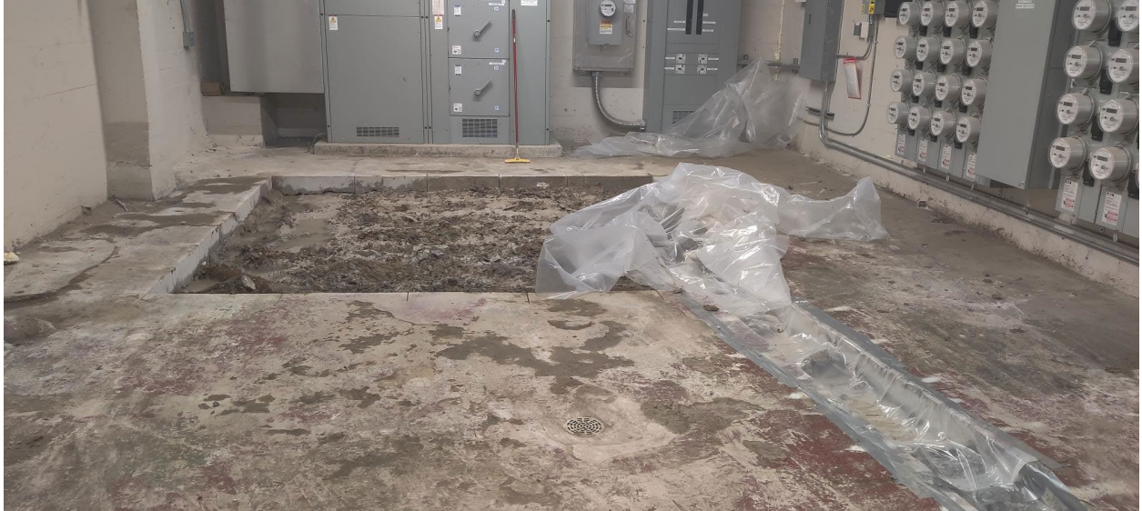
Picture 4: Concrete cut and removed from N Mechanical Room
