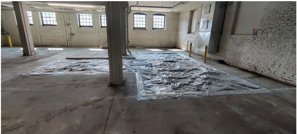
Picture 5: Concrete cut and removed from SW Garage
