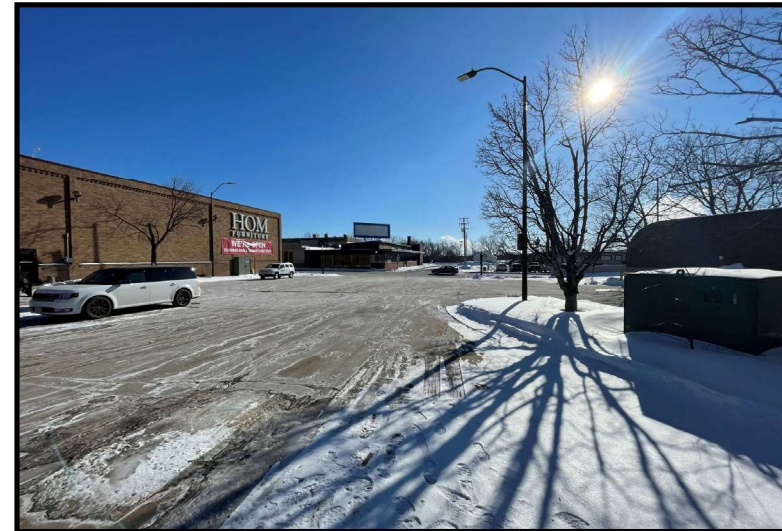
Concrete cap on 2nd Street right-of-way and Outlot 3 (01/31/2023)
