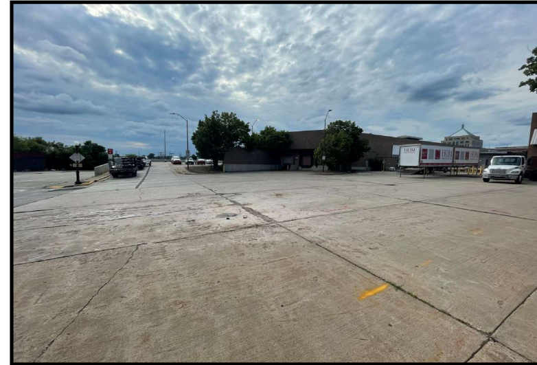
Concrete cap on 2nd Street right-of-way and Lot 1 (07/26/2022)
