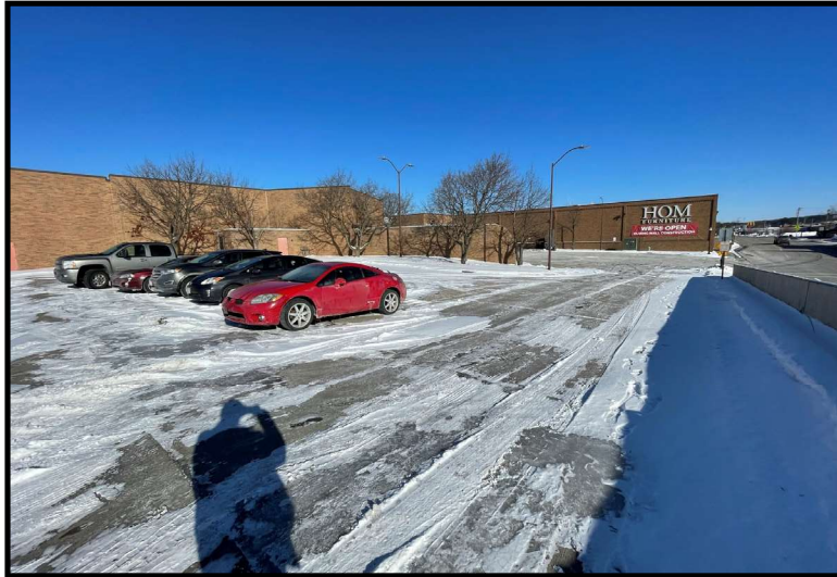
Concrete cap on Lot 1 (01/31/2023)
