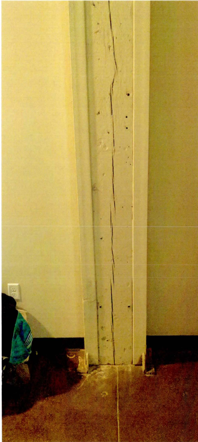
Picture 6: Unit 1014 - Wooden Pillar in the bedroom
