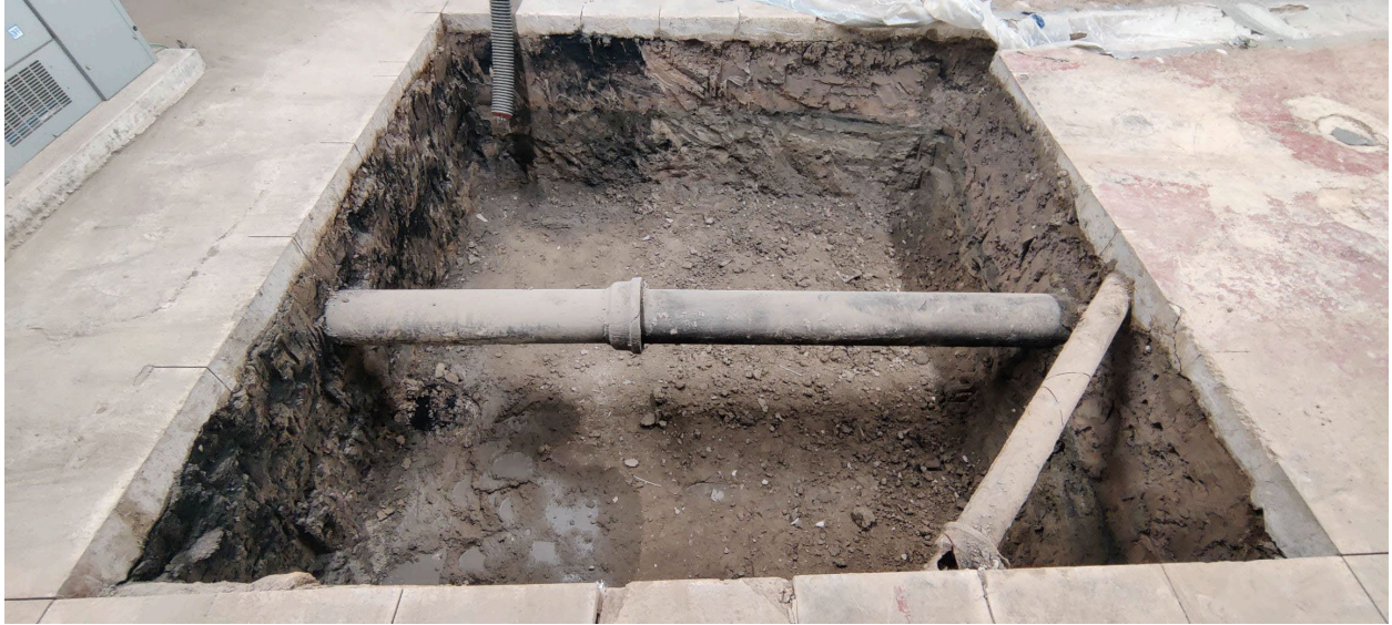
Picture 1 – N Mechanical Room Excavated Area
