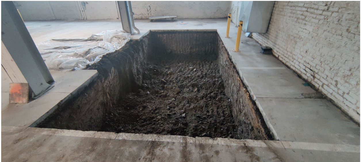
Picture 2 – SW Garage Excavated Area
