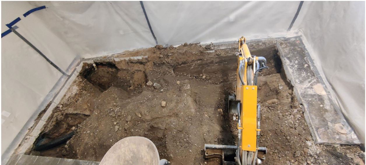
Picture 8 – Unit 1045 Living Room Area Excavation in Progress
