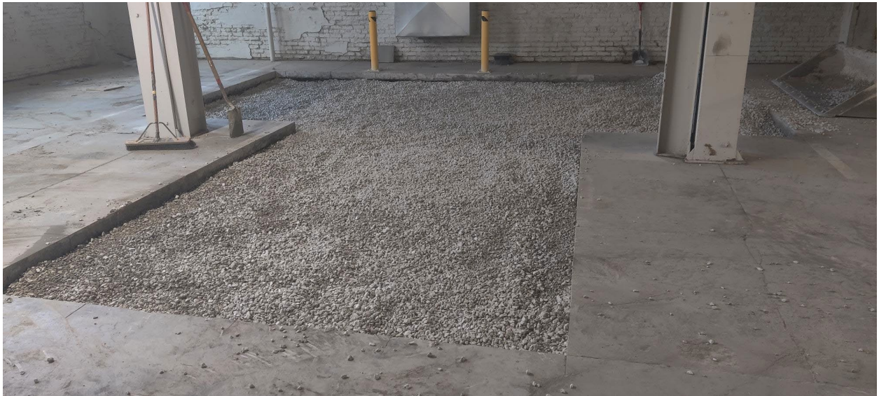
Picture 4 – SW Garage Area
