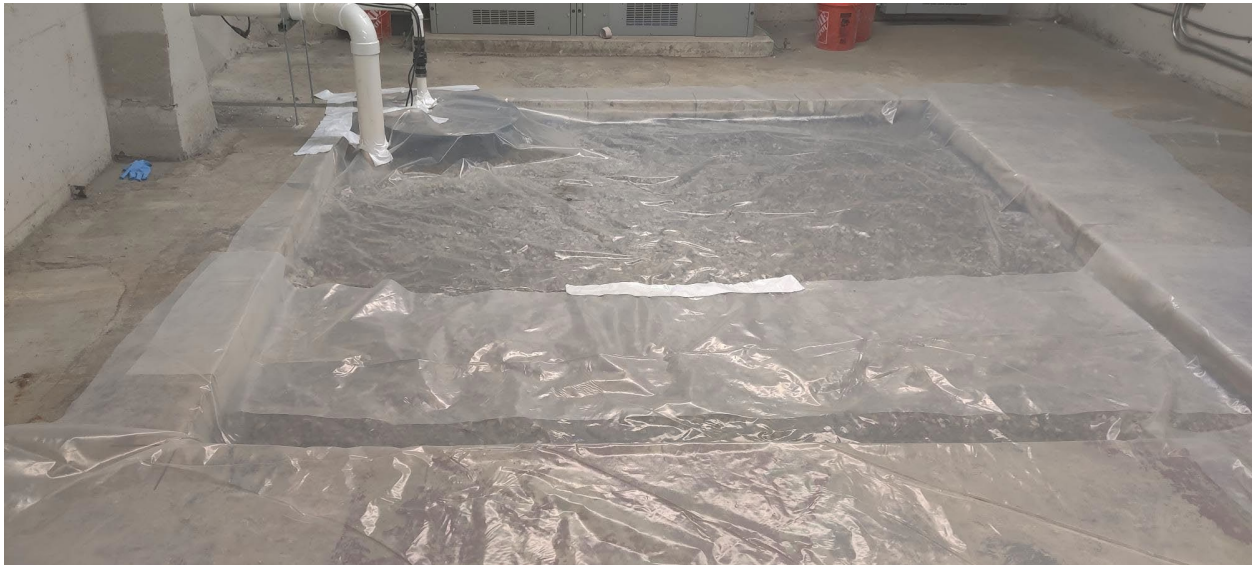
Picture 2 – N Mechanical Room Excavated Area
