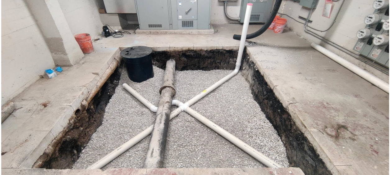
Picture 1 – N Mechanical Room Excavated Area
