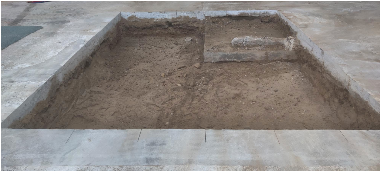
Picture 6 – BB2 Gym Area
