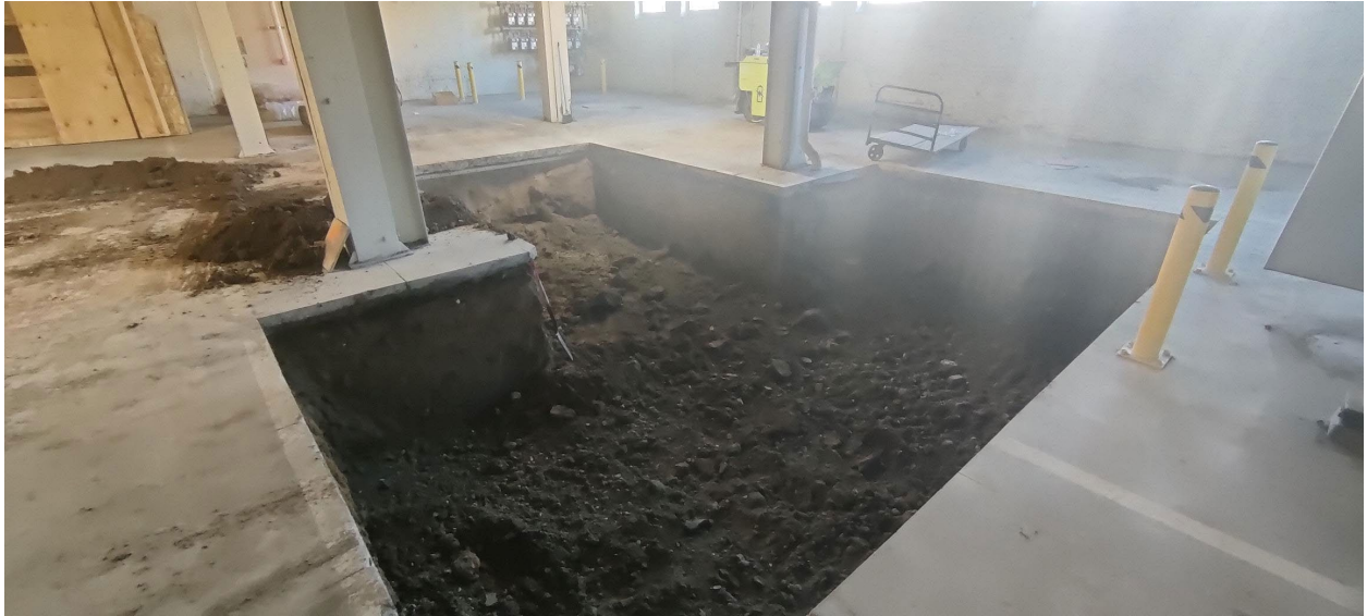
Picture 3 – SW Garage Area
