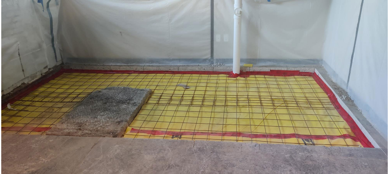
Picture 1 – Excavated Area in Unit 1044 with Extraction Point
