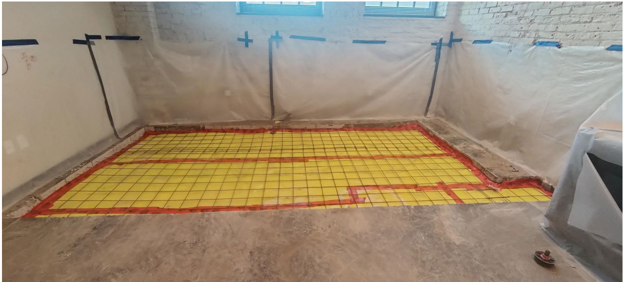
Picture 2 – Excavated Area in Unit 1045 – Living Room
