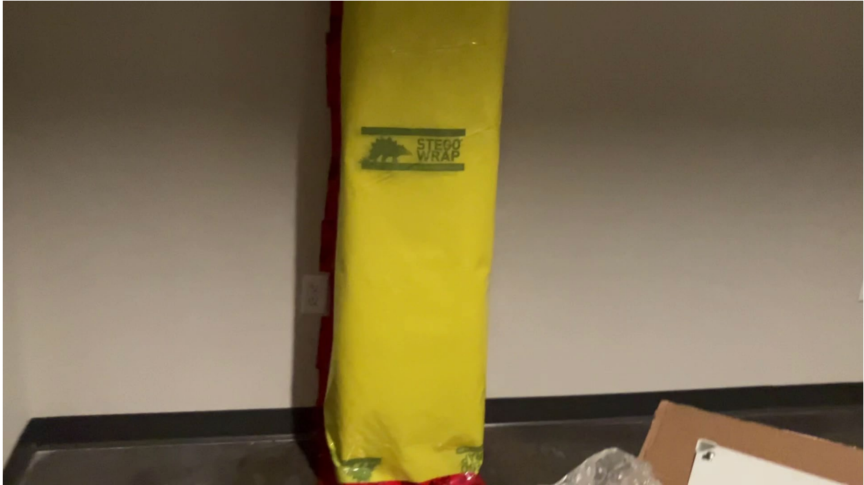
Picture 1. Vapor Barrier Sealed Column located in the bedroom of Unit 1043
