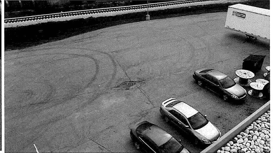
Photograph 22 - View southeast of east loading dock
