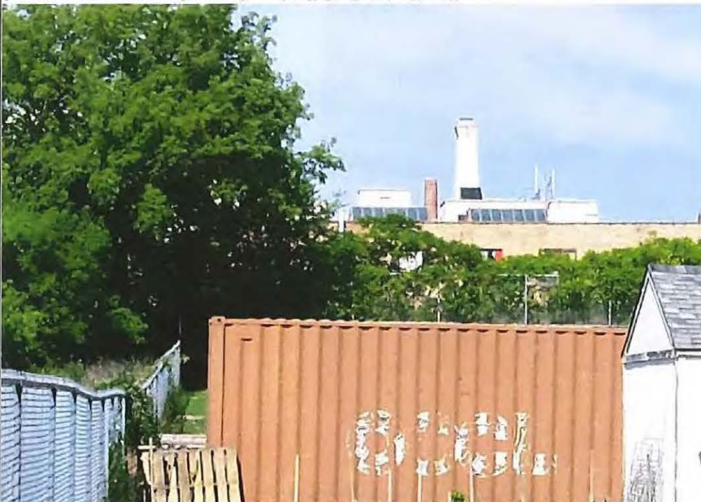
Title: Wisconsin Industries Pension Plan & Trust/02-41-263675/July 20, 2016/East side depressurization system stack, middle of photo.
