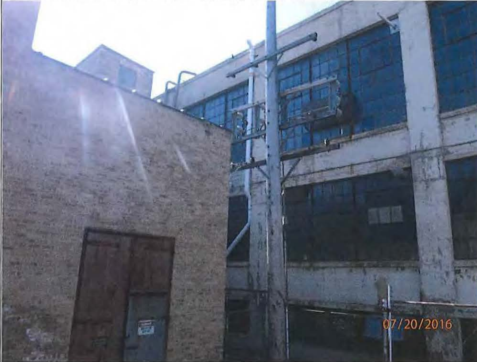
Title: Wisconsin Industries Pension Plan & Trust/02-41-263675/July 20, 2016/West side depressurization system stack.
