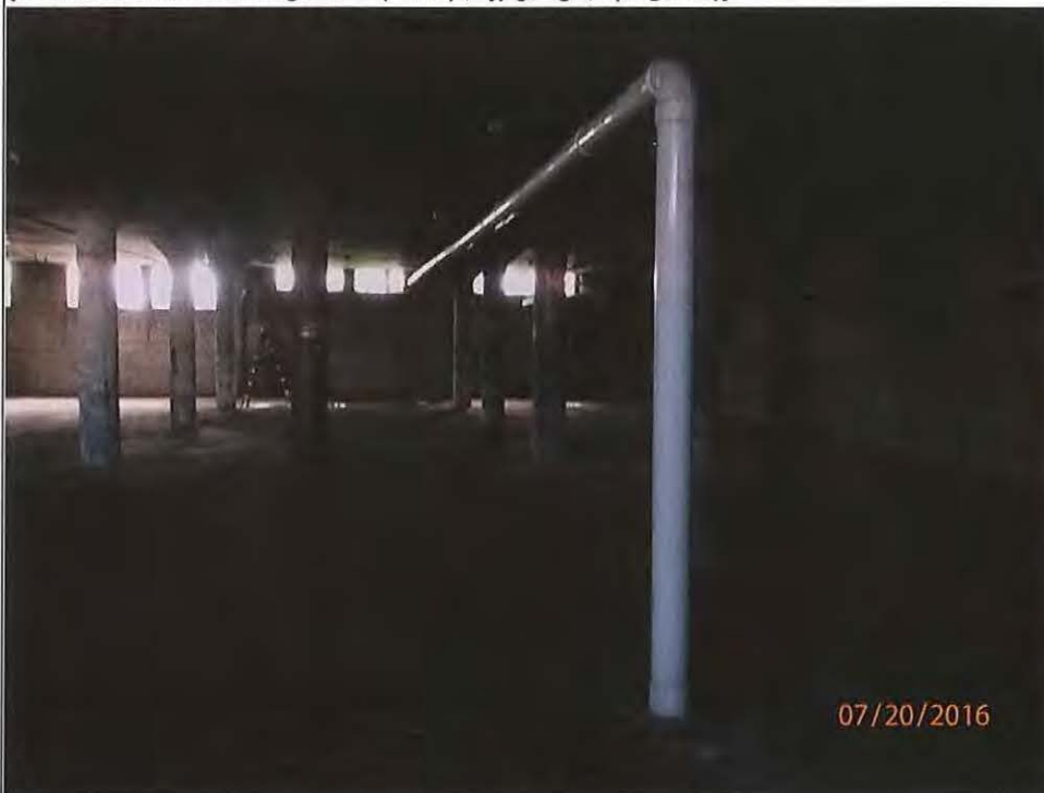
Title: Wisconsin Industries Pension Plan & Trust/02-41-263675/July 20, 2016/East side depressurization system.
