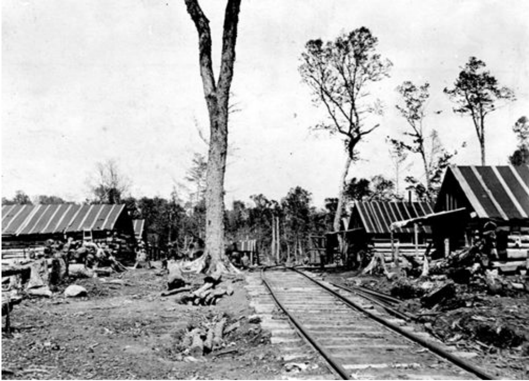
Figure 8. The Brown Brothers logging camp sat on the Wisconsin side of the state border immediately north of Spring Lake. The camp operated from 1900 to 1909. The photo was shot during summer, 1908 (Janet Vineyard).
