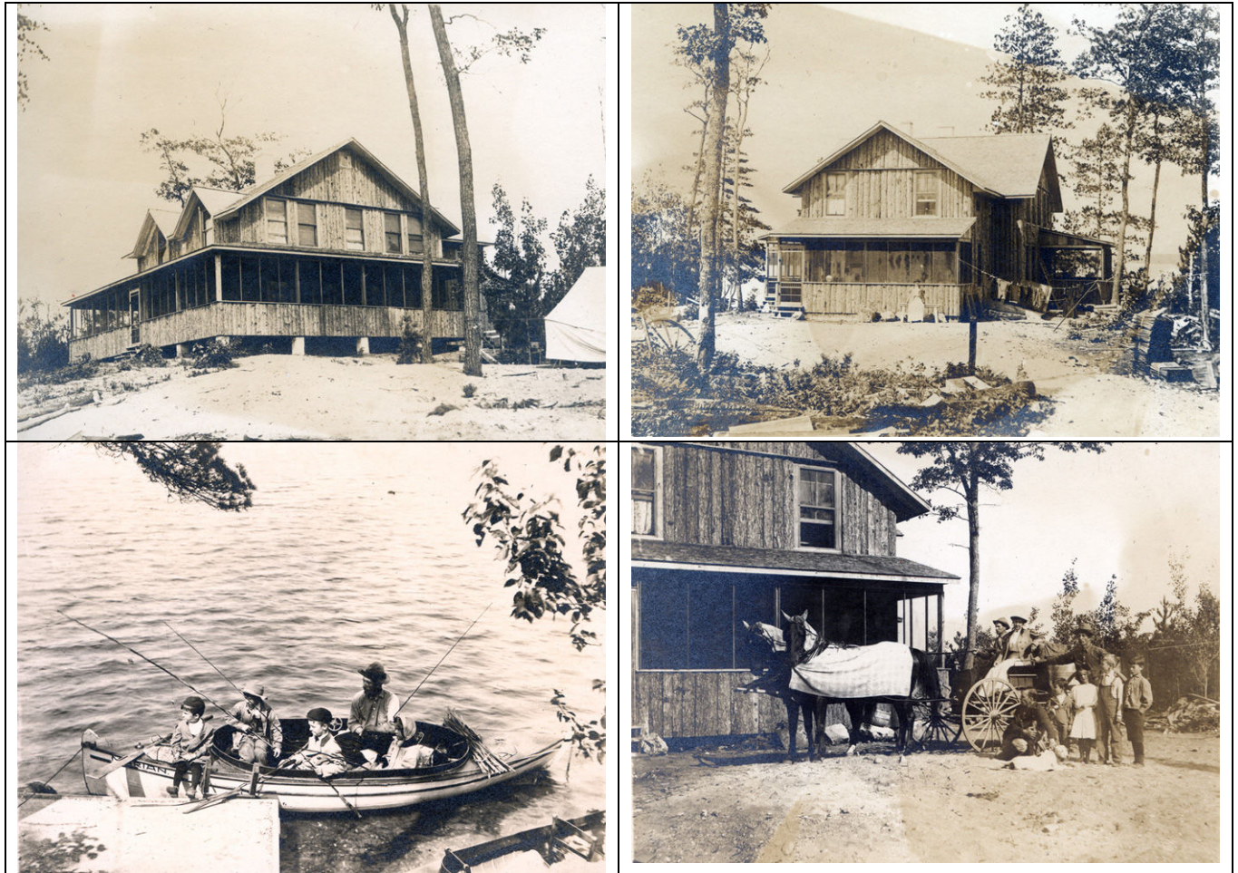
Figure 13. Images of the Lee Barber house and family. The house was completed during the summer of 1908, and the photographs were shot in August, 1908 (Paul McLeod).
