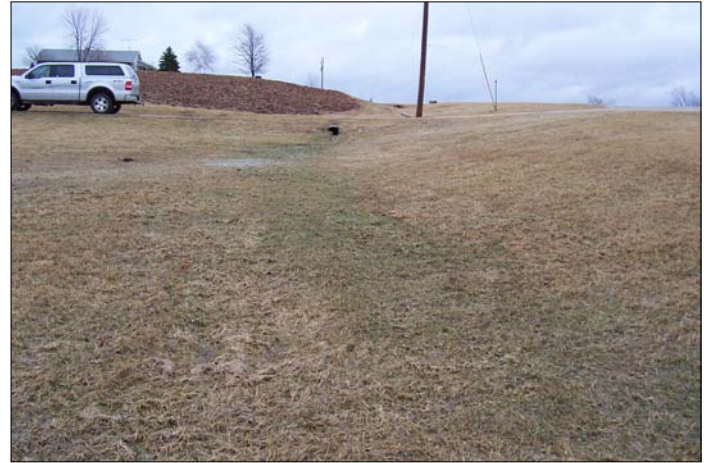
Photo 2: First Driveway Culvert
