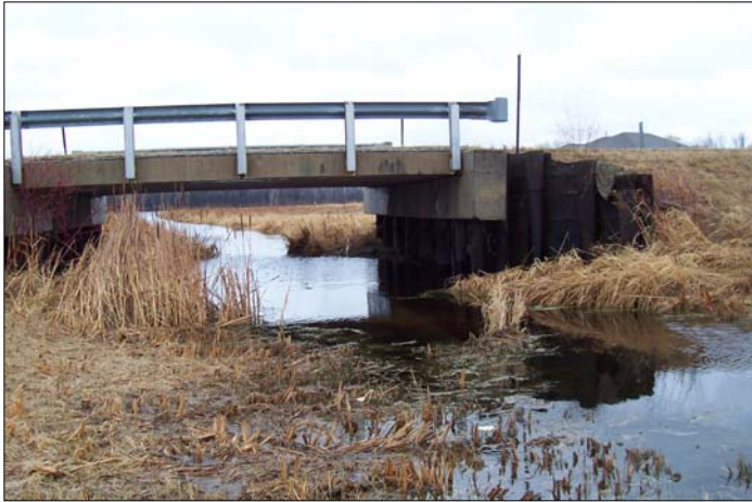
Photo 1: Bridge Sampling Location
