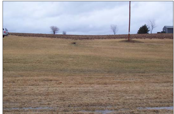
Photo 4: Second Driveway Culvert
