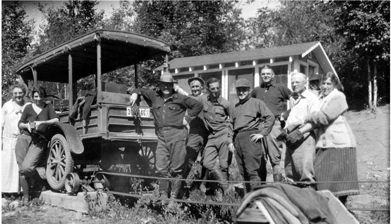
Figure 20. Ross Woodhull (in cowboy hat) and Nick Lowenstine (in baseball cap) began inviting Valparaiso, Indiana friends up to their houses every summer beginning in the early 1920s. The photo, dating to around 1923, may have been shot during the construction of the Lowenstine house (Jane Lohmeyer).
