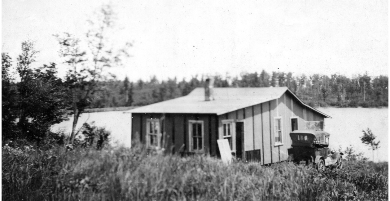
Figure 26. The Torres cabin at the west end of Black Oak Lake. The Torres family acquired the cabin from Walter Dickman in 1922, and while the cabin was rebuilt in the 1940s, the family still owns the property (Ed Torres).
