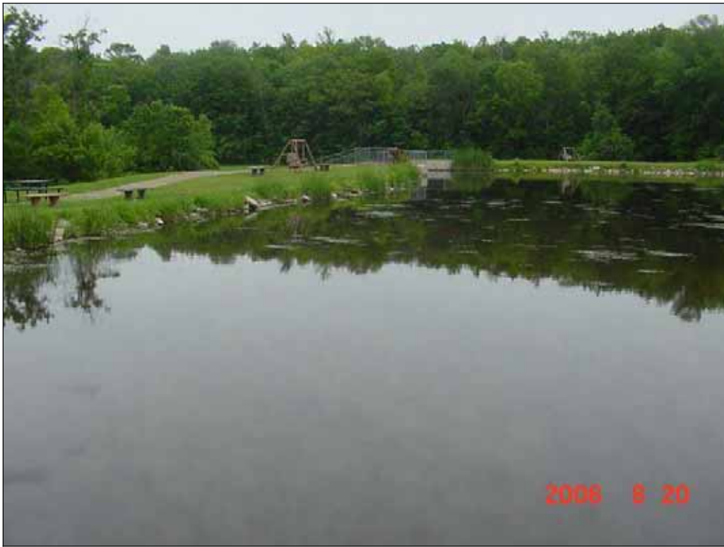
Site 8 - Glenbeulah Dam
