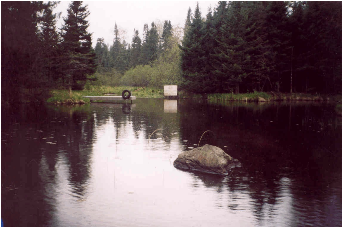
Figure 11. Outlet area, May 2004.
