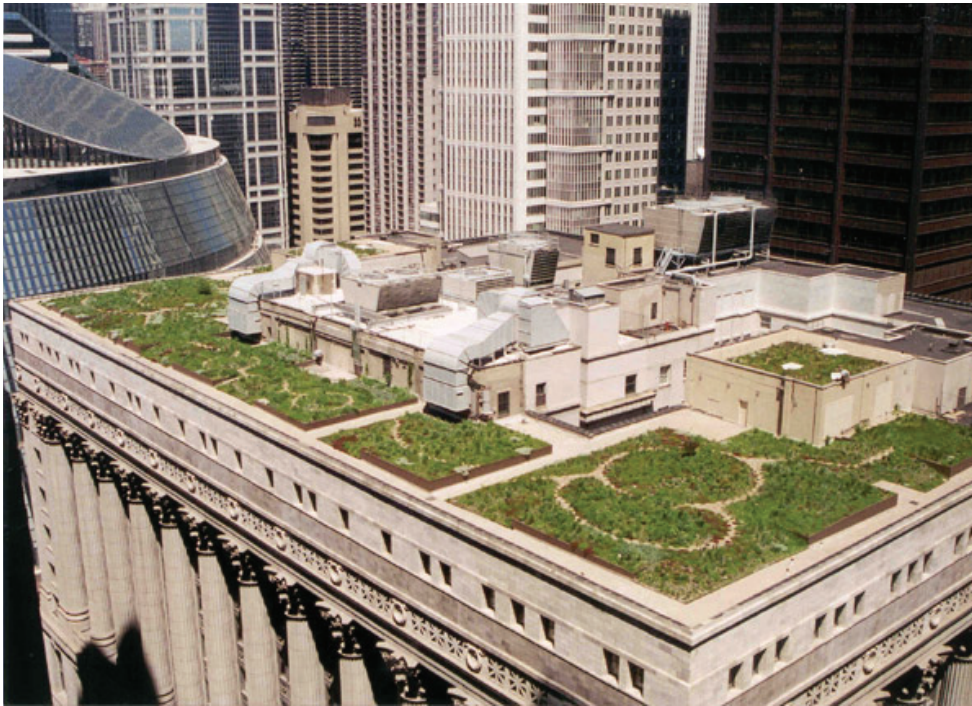
Figure 6.8. Green roof on Chicago City Hall (from Chicago Department of Environment, 2007).
