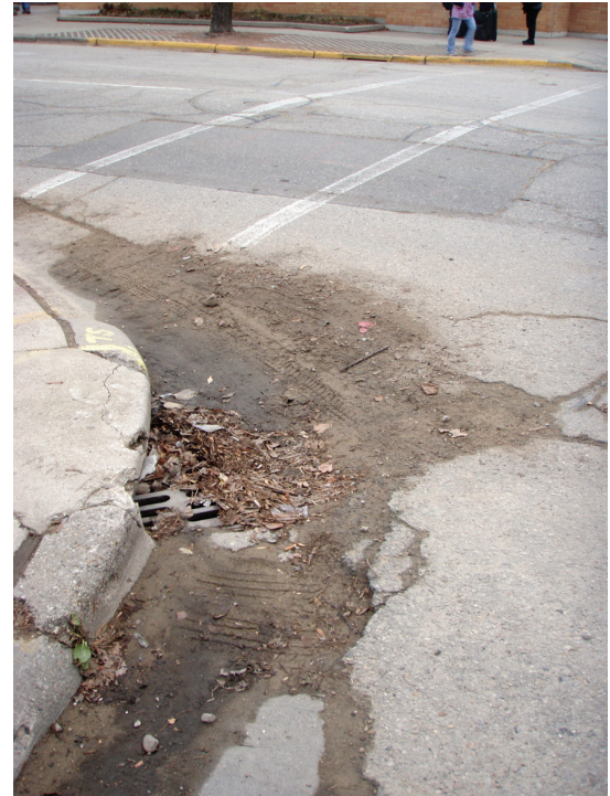
Figure 6.2. Sediment clogging a storm drain adjacent to a construction site in the Monona Bay watershed.
