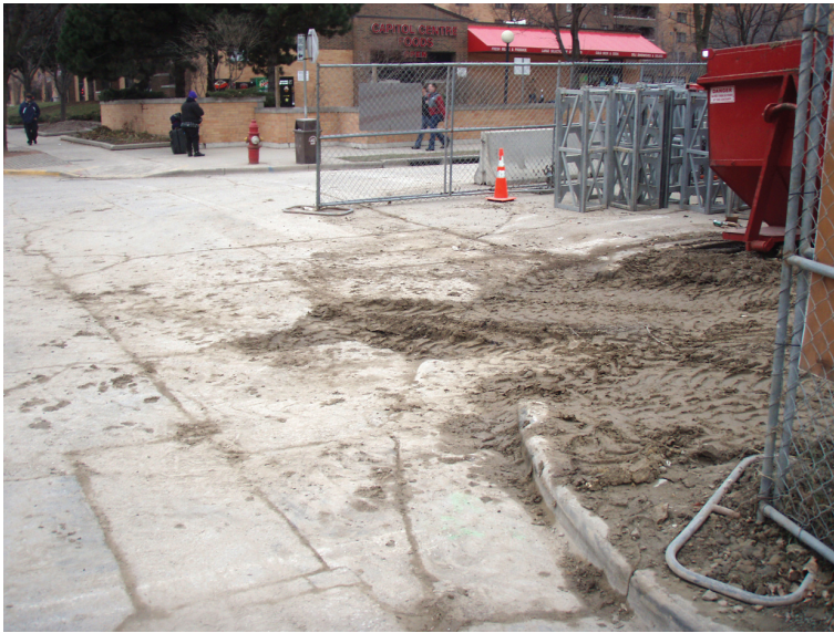
Figure 6.1. Sediment tracked onto street from equipment at a construction site in the Monona Bay watershed.
