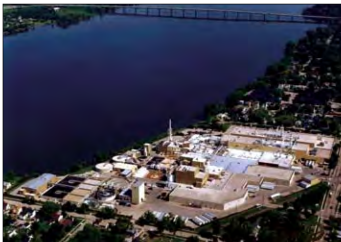
SCA’s Menasha plant manufactures paper for napkins, paper towels and other products using 100% pre- and post-consumer recycled fiber. Photo courtesy SCA Tissue.
