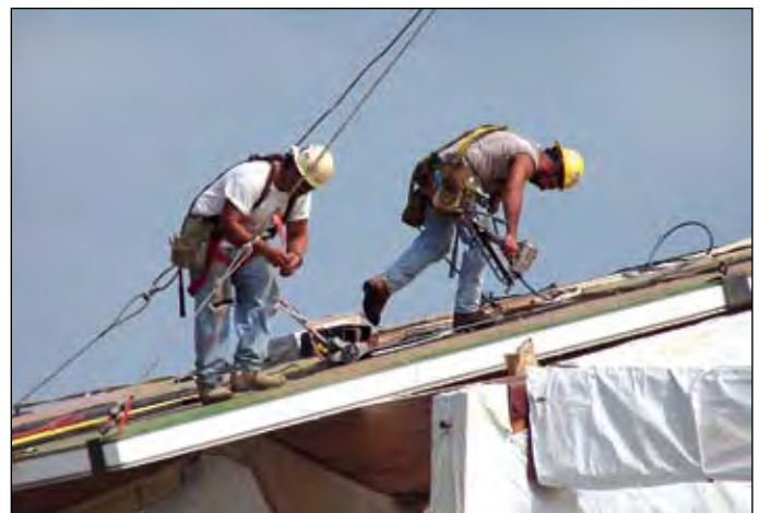
Workers install Structural Insulated Panels (SIPs), made from rigid EPS foam sandwiched between two laminated board layers, on a roof. Photo courtesy Plymouth Foam.
