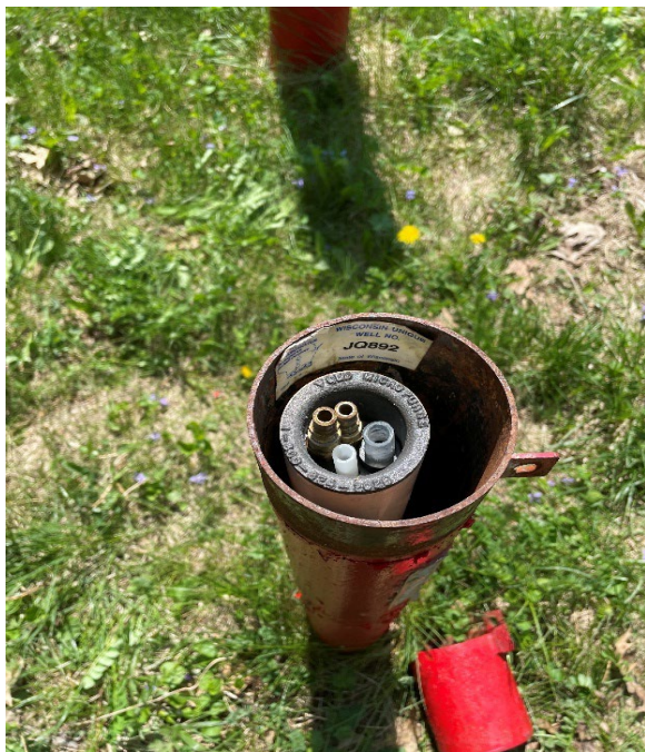
Photo 9: WUWN sticker displayed on inside of groundwater monitoring well protective cover pipe.
