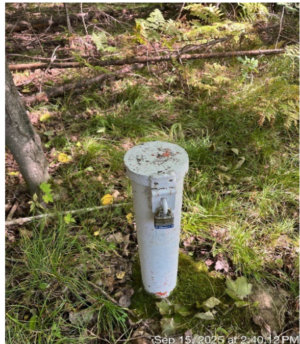
Photo 2: Protective cover pipe with lock.
