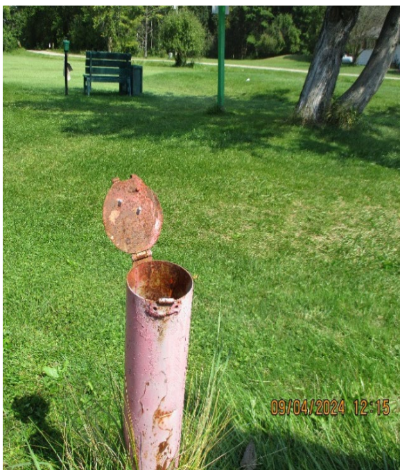
Photo 3: Protective cover pipe without lock.
