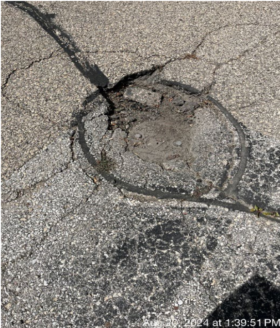
Photo 1: Protective cover pipe for flush-mounted groundwater monitoring well.
