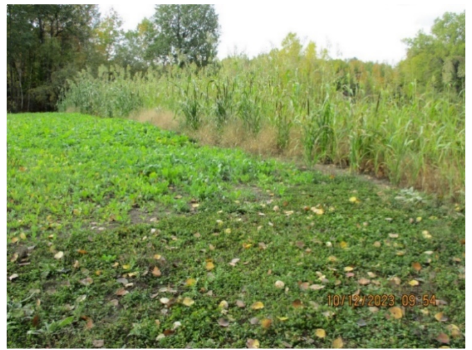
Photo 8: Example of landfill cover planted with crops, which is improper vegetation on landfill cover.
