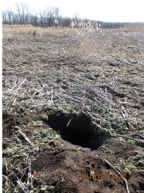
Photo 4: Animal borrow hole on landfill cover.
