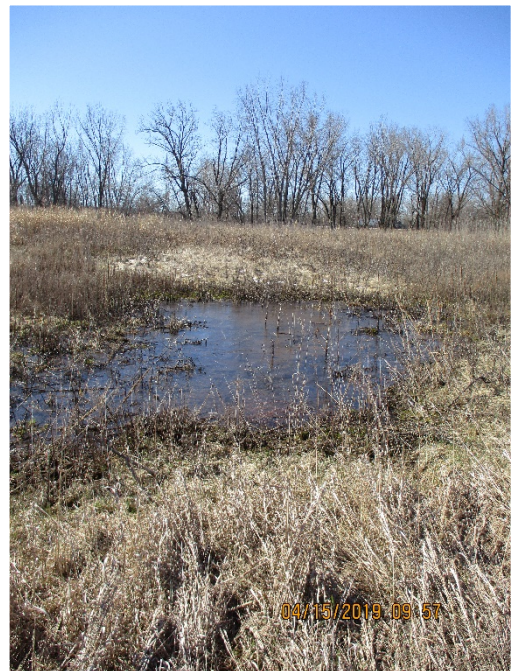
Photo 13: Example of landfill surface with ponding water.
