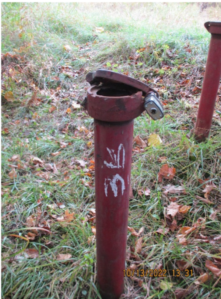
Photo 20: Lid on outer metal protective casing that can be opened even with a lock installed.
