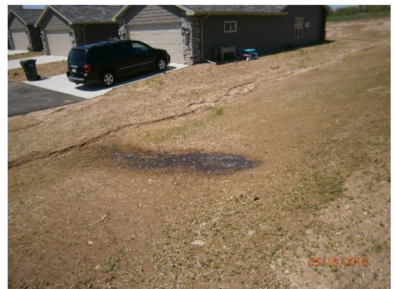
Photos 31: Leachate seep on side slope of landfill.
