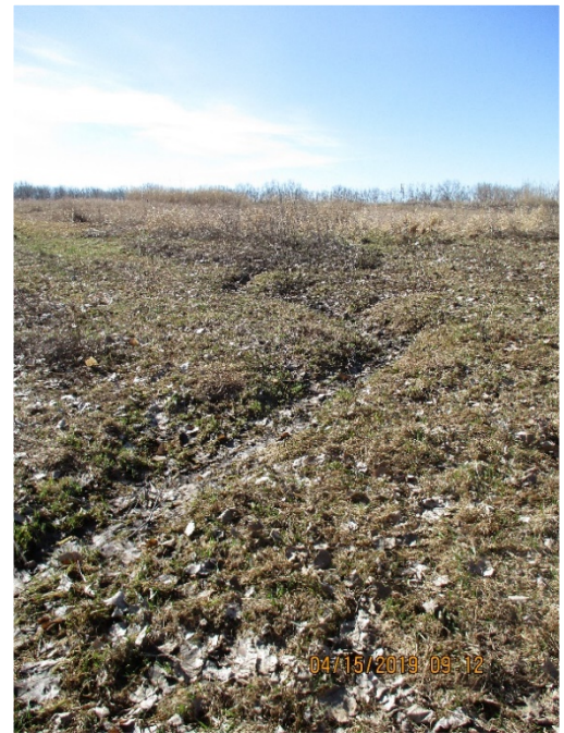
Photo 1: Gully type erosion on landfill cover.
