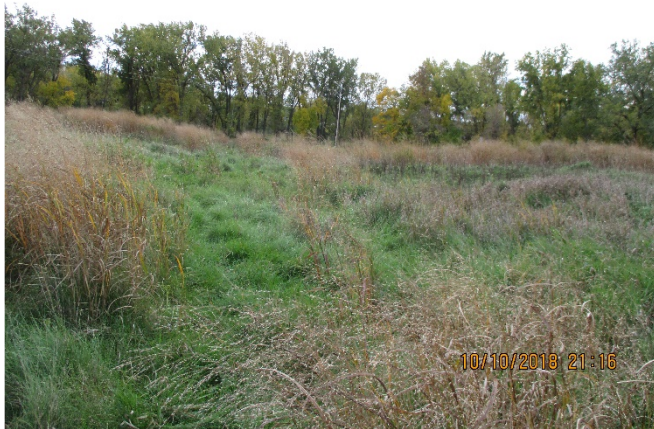
Photo 12: Example of uneven landfill surface that needs regrading if water begins to accumulate in the lower area.
