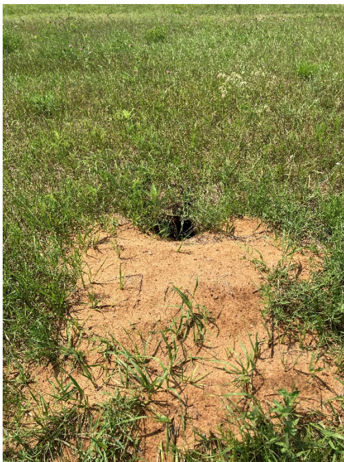
Photo 3: Animal borrow hole on landfill cover.3
