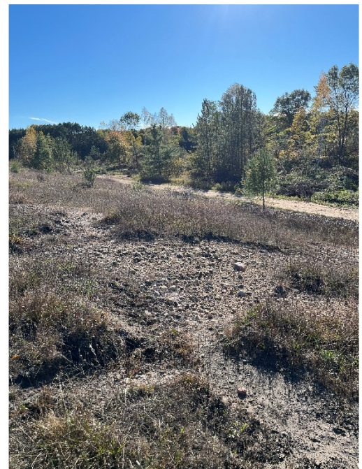
Photo 2: Erosion on side slope of a landfill cover.
