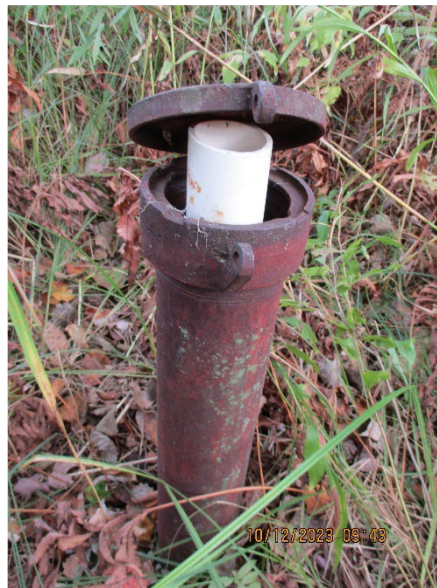
Photo 21: Groundwater monitoring well that cannot be locked because the inner well casing has raised above the top of the outer metal protective casing.
