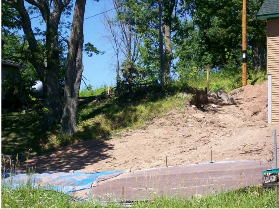
Erosion near the Ward Lake shoreline
