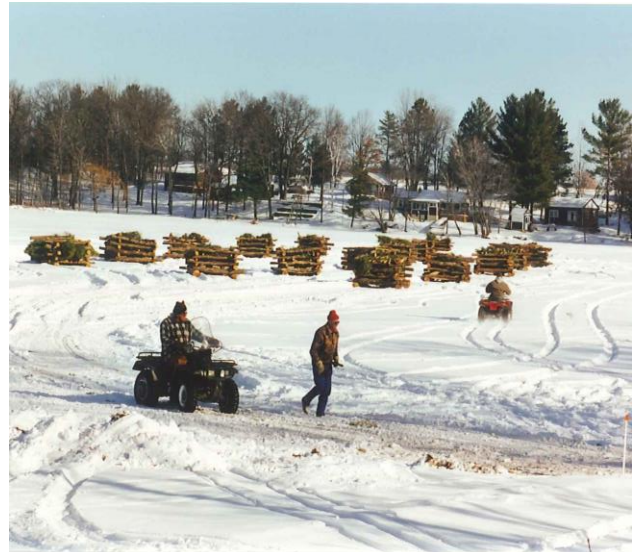
Figure 6. Fish cribs being installed on Amacoy Lake during the winter.
