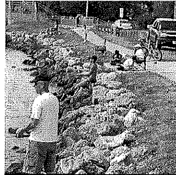
Riprap is a common shore protection practice
