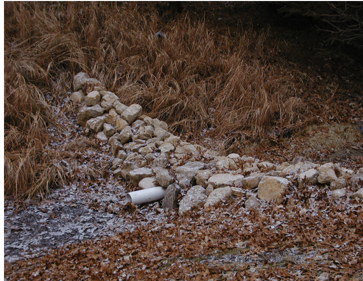
Leyton Lane Check Dam
