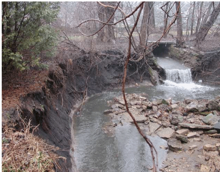
Manitou Way Storm Sewer Outfall
