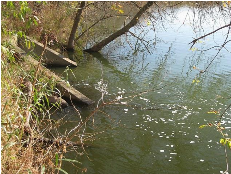
Figure 11. Side-view of outfall and concrete structure supporting high exit velocity.
