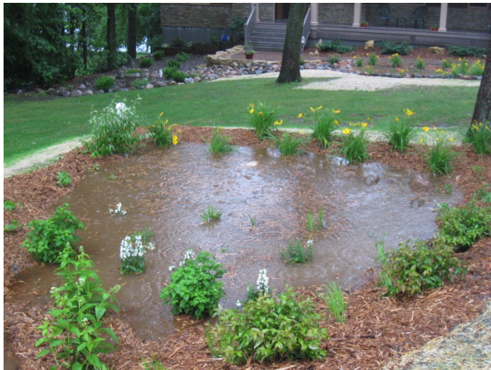
Figure 21. Rain Gardens Collect and Infiltrate Runoff Water (photo by Steve Palmer)
