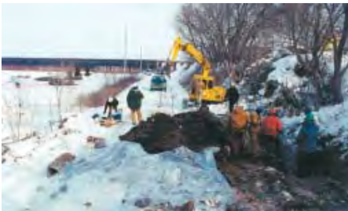
Cleanup of Ashland Coal Tar Site seep.
