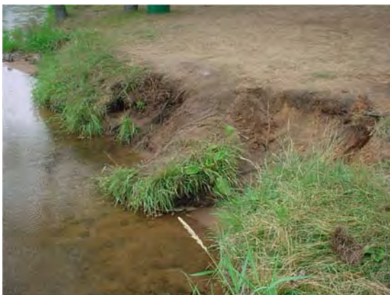
Figure 1: Shoreline in need of restoration (photo: Tom Littwin)
