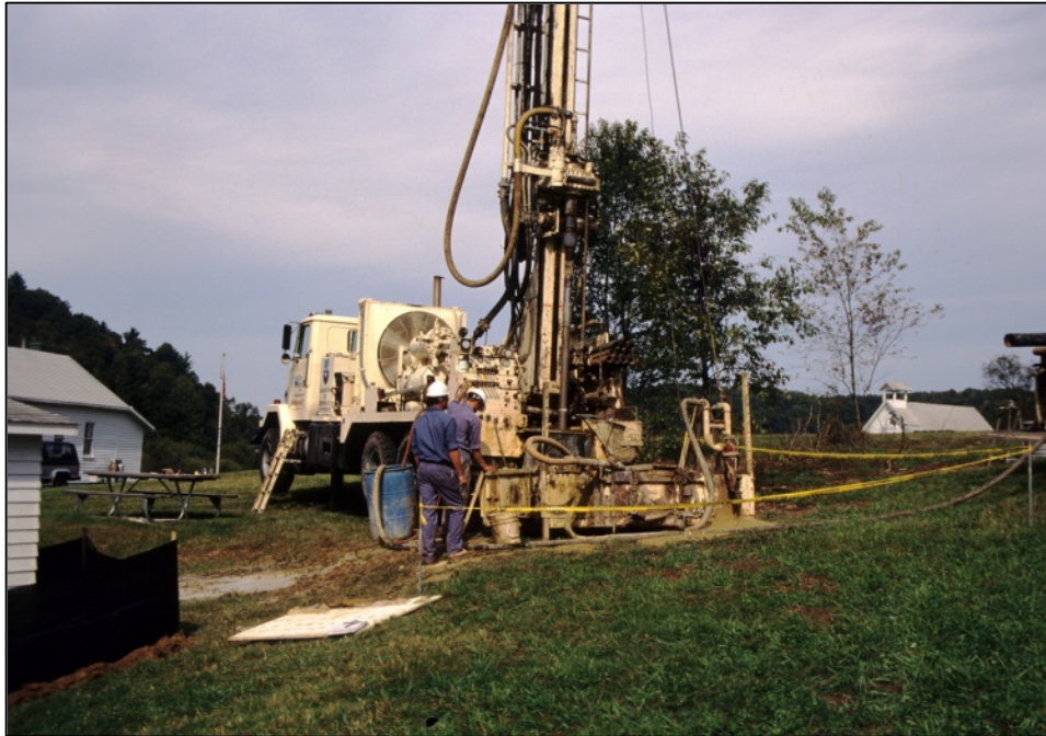
Drilling a well on rural property.
