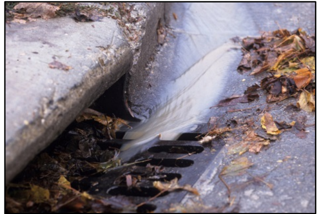
Stormwater drain receiving runoff
