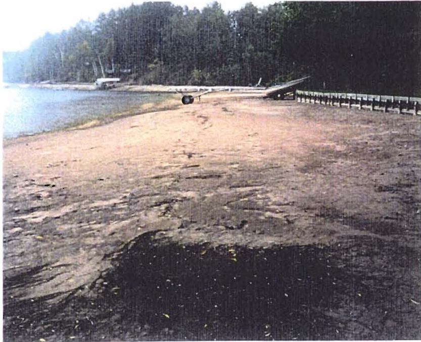
Townsend Flowage, 1993, drained to repair dam.
