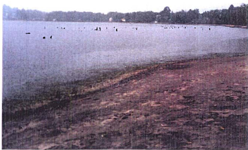
Townsend Flowage, -1993, drained to repair dam.
