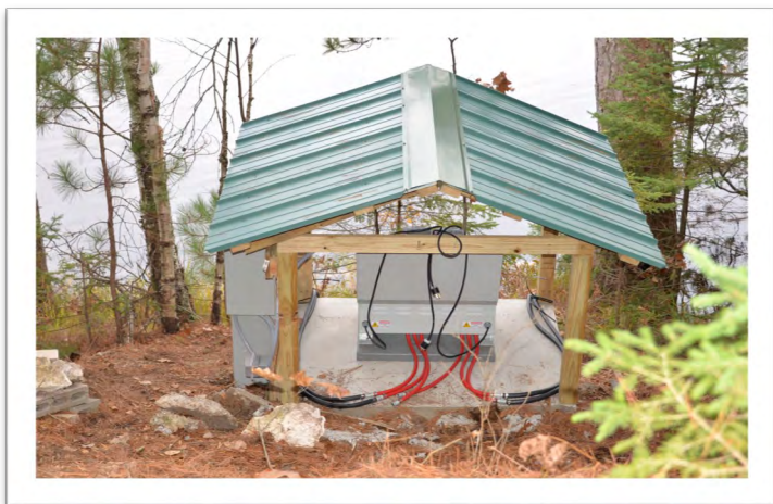
New Long Lake aerator during installation
