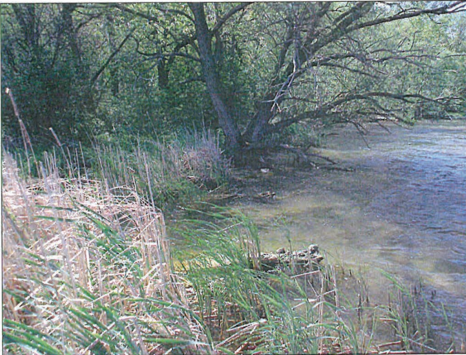
Photo #8 – Hooker Lake Dam (May 20, 2009)
