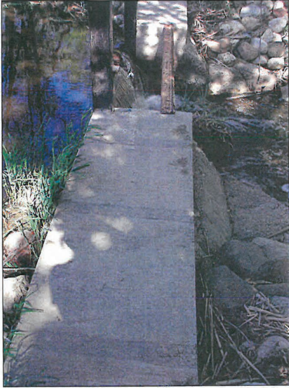
Photo #1 – Bryzek Dam (May 20, 2009)
