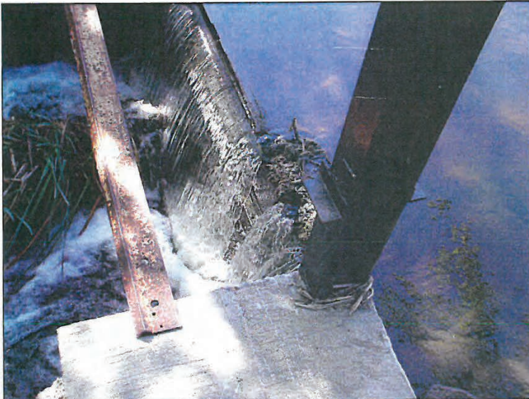
Photo #2 – Bryzek Dam (May 20, 2009)
