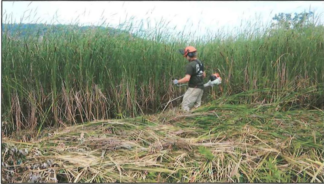
August 2016. A worker from Integrated Restorations using a Stihl weed cutter to cut hybrid cattail. The cut stems were then treated with imazapyr herbicide.
