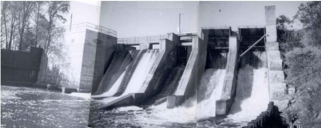
Figure 9. The Black Brook Dam
