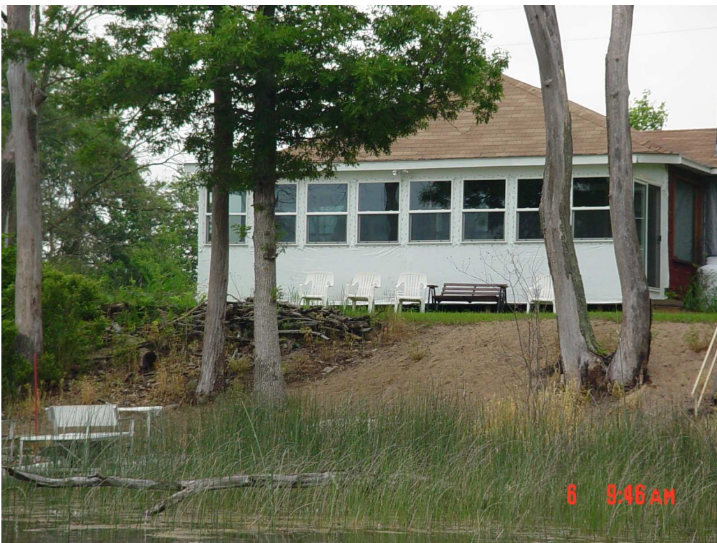
Figure 13: Example of Inadequate Vegetative Buffer
